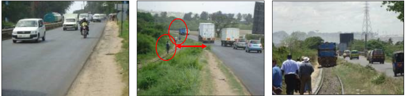
Sections of Makupa Causeway Section (Note the Safety Risks)
