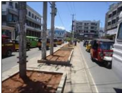
City Centre Overhead Lines
