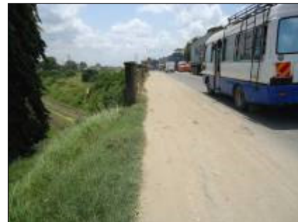
View of ROB at Changamwe
