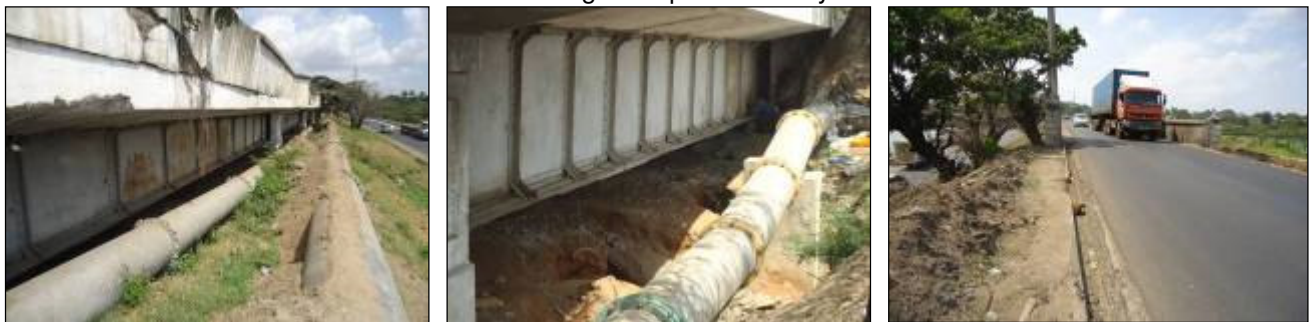
Existing Makupa Causeway Bridge
