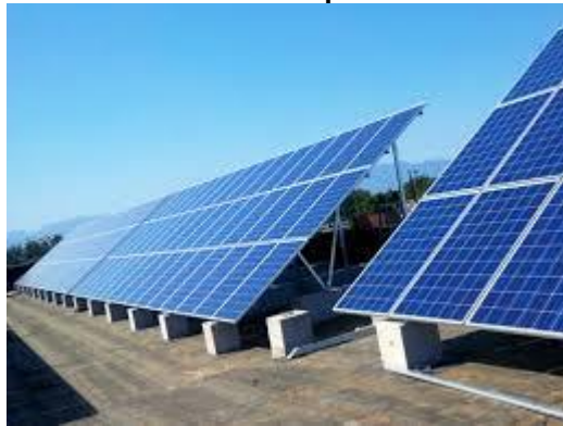
Figure 3.5: 'Solid state' silicon solar panels with ballast foundations
