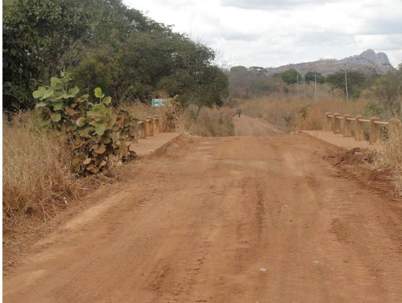
Figure 2: A typical rural road and bridge in the project area (Ribau district)
