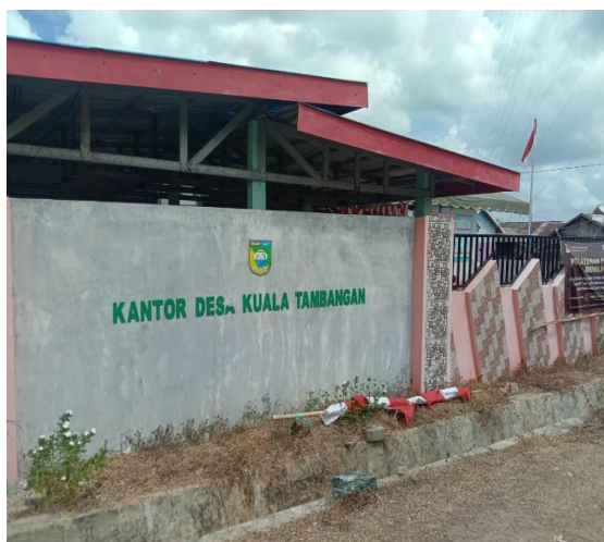
Kuala Tambangan Village Office
