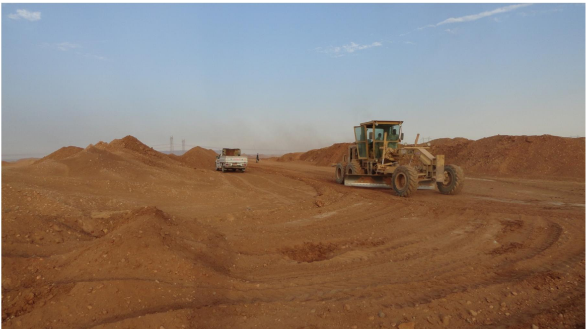
Figure 19: Road construction on site (Fall 2015)
