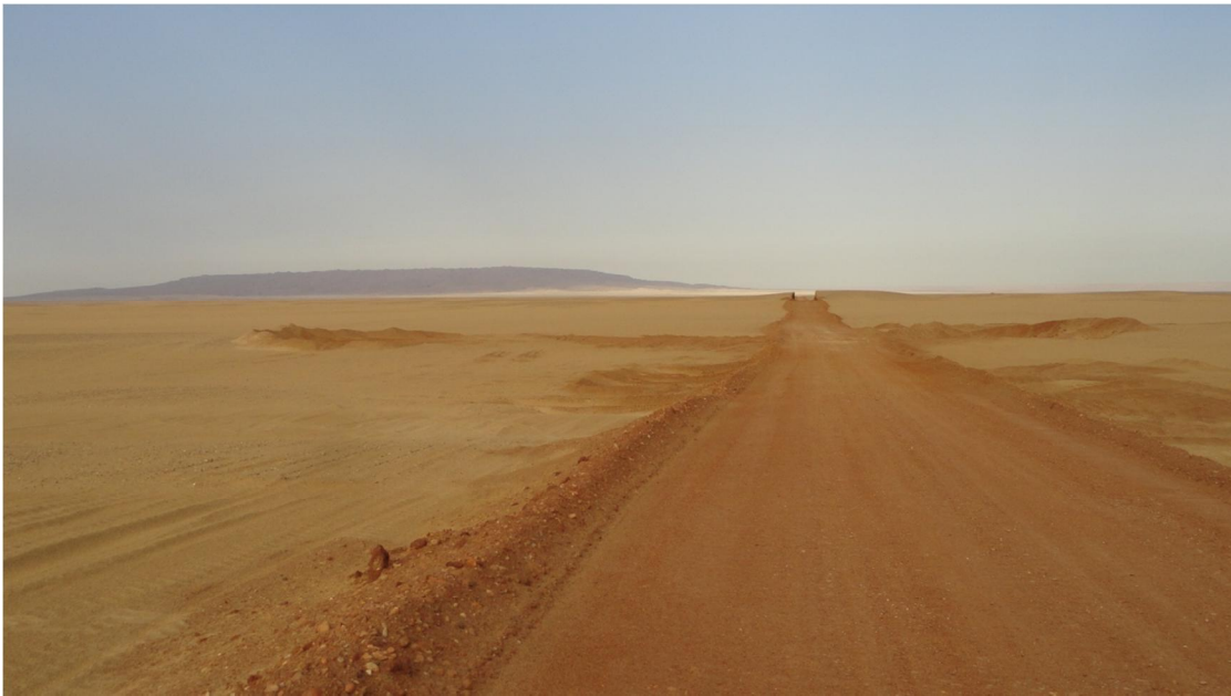
Figure 9: View to the west, along a site service road (under construction)
