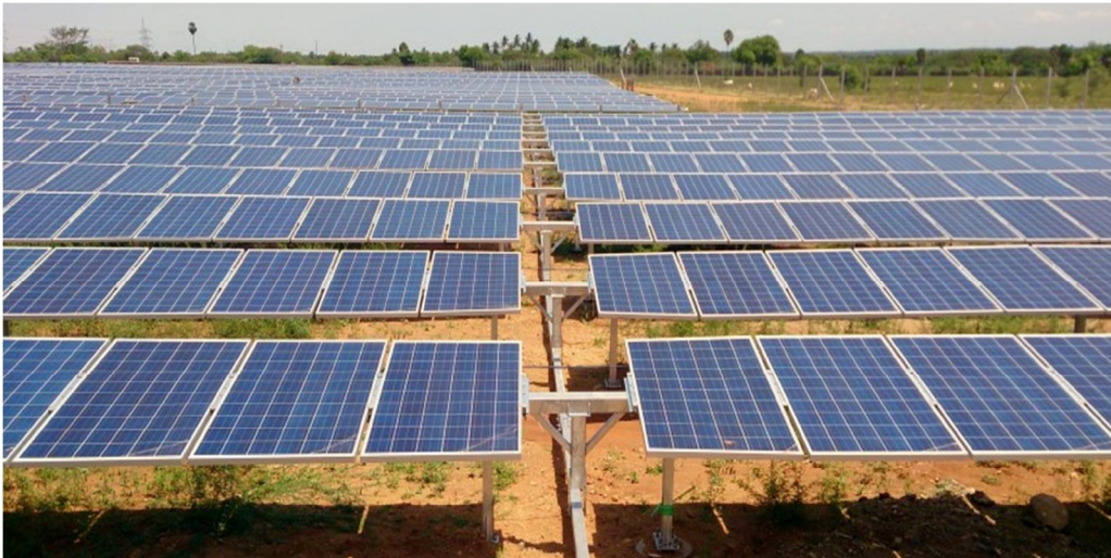
Figure 29: Single axis tracker system
