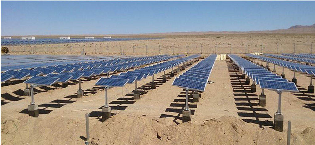
Figure 28: Tilted mounting of panels on fixed frames (Sonnedix Atacama)
