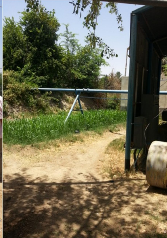
Figure 63: Existing Benban village intake
