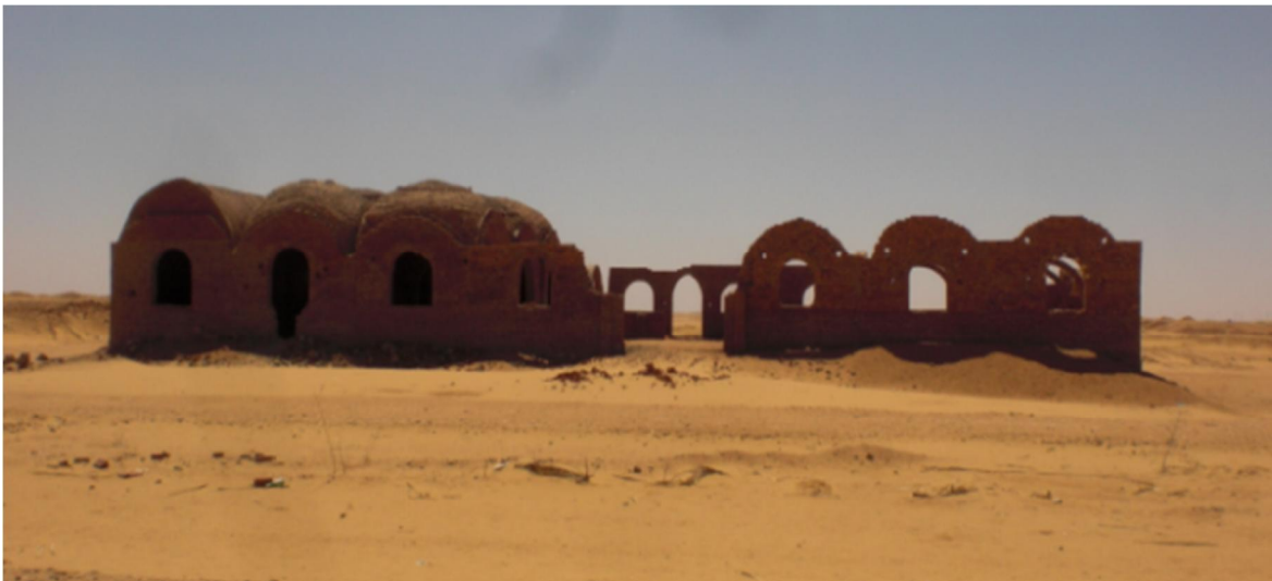
Figure 6: Illegal buildings near Aswan – Luxor Highway (close to the Benban village turnoff).
