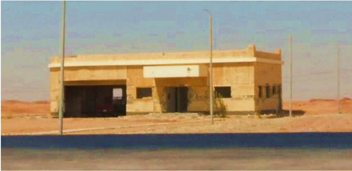
Figure 5: Abandoned ambulance station near Aswan – Luxor Highway (close to the Benban village turnoff).
