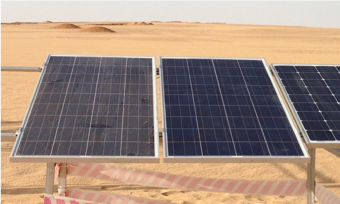
Figure 81: Trial panels at Benban
