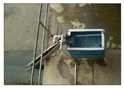
Figure 17 shows the trap system with ramp leading to a holding tank and piped water supply installed at Waitaki Dam, New Zealand. The ramp can be lined with bristles, gravel or a drainage product called Miradrain or Cordrain (Patterson & Boubee 2010). The optimum slope is about 15 degrees.
