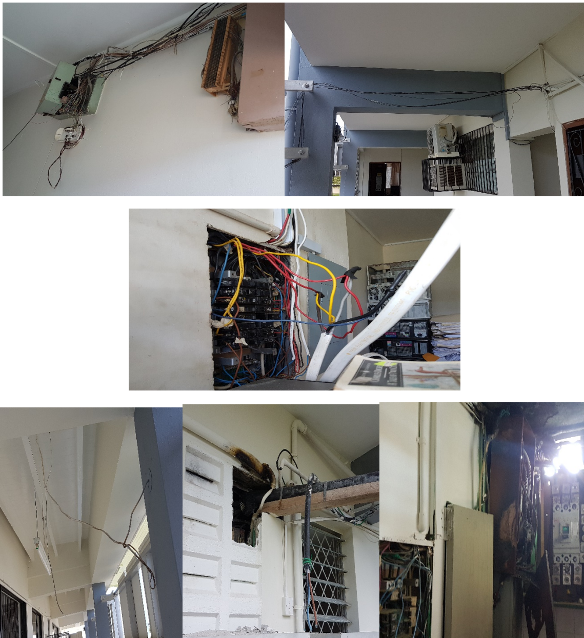
Exposed electrical wires, open face panel and low hanging wires at the Faculty of Health Sciences
