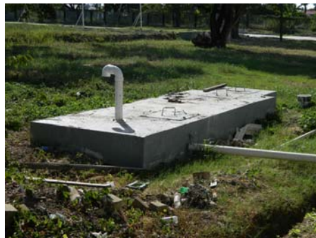
Septic tank constructed for the Faculty of Technology
