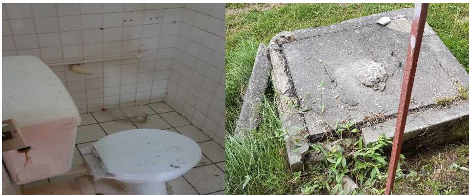
Unsanitary toilet and partially decaying septic system
