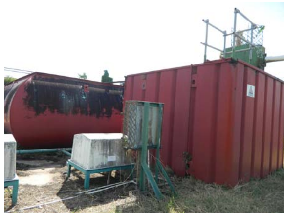
Primary Settling Tank and the Aeration Tank at the Turkeyen Campus, University of Guyana.
