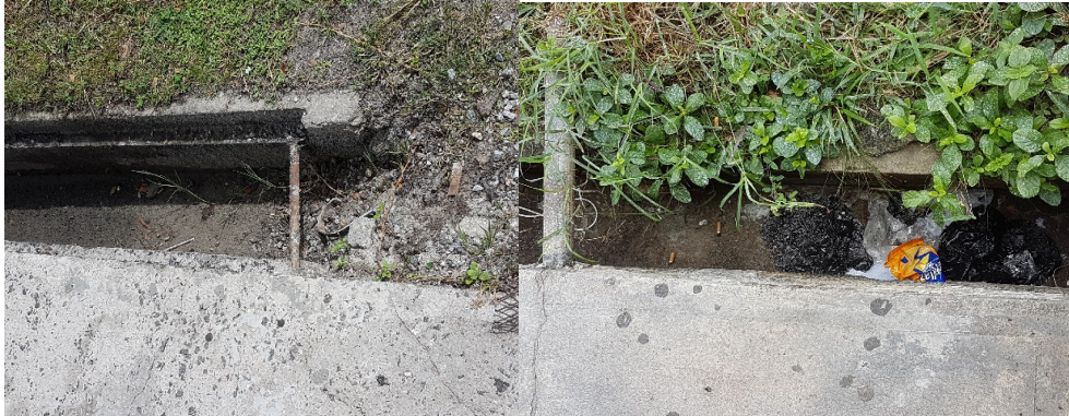
Garbage Filled and incomplete drains
