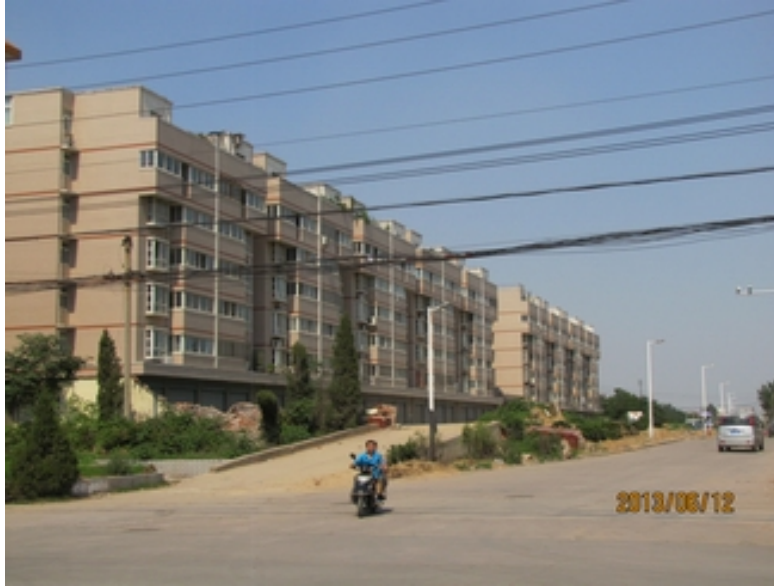
Fig.7.2-8 Photo of current status of north extension of Changxing Road (III) Comparison of Line Schemes
