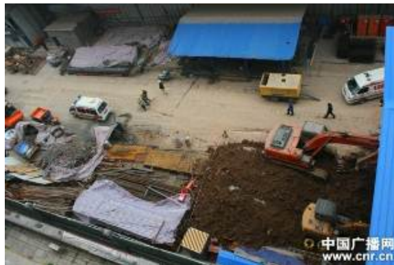
Site of Landslide Accident in No. 3 Subway in Xi'an
