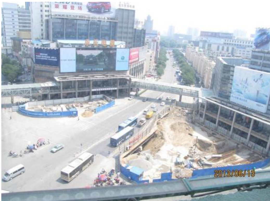
Figure 5.10-6 Erqi Square circular corridor
