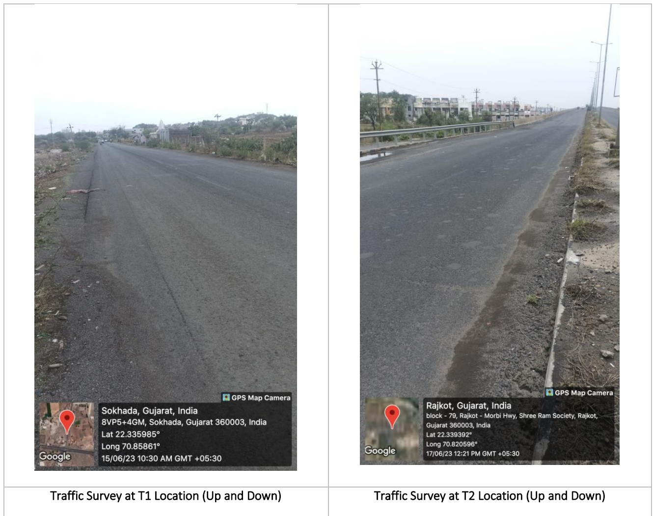
Figure 5-21 Traffic Survey Monitoring conducted in Study Area
