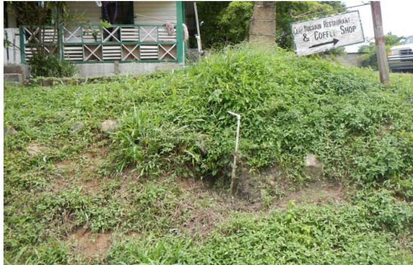
Figure 5.2: Exposed Water Infrastructure along ROW.
