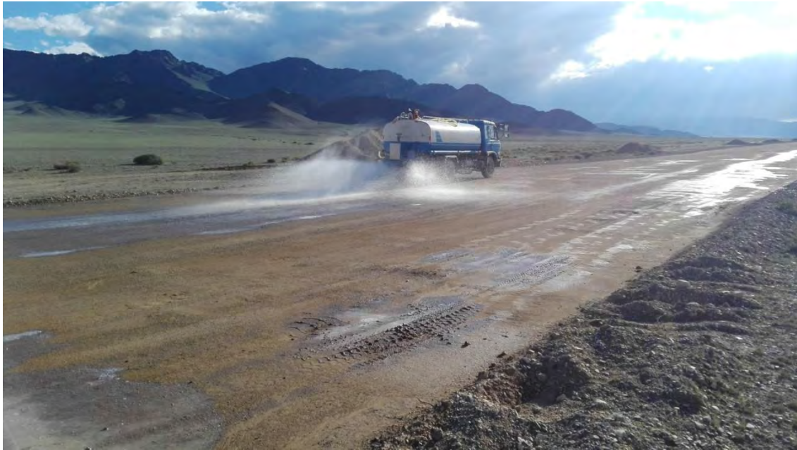
Figure 6. Water spray truck, CW1-1
