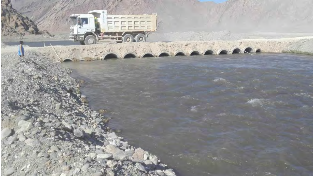
Figure 15: A deviation road embankment over the Buyant river
