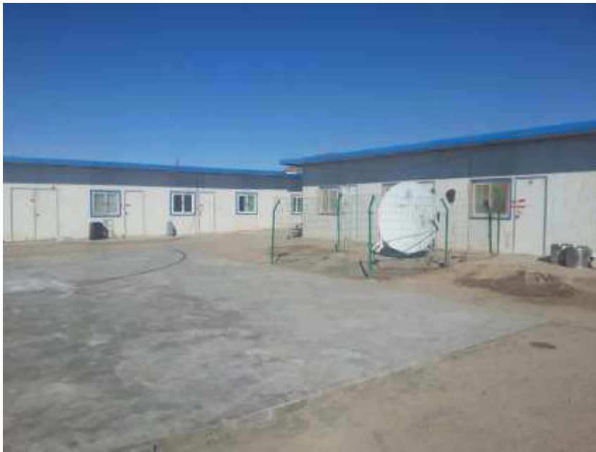
Figure 8: Workers' accomodation at the Package I Main camp.
