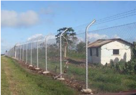
Figure 11 South western perimeter fence with no concrete edge beams
