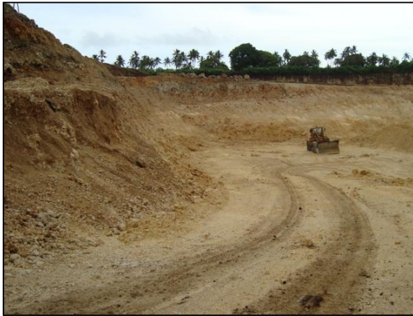
Figure 7 Quarry Site Q2 in operation
