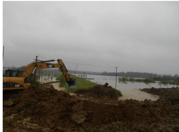
Cutting through the dam Paljuvi Viš 1
