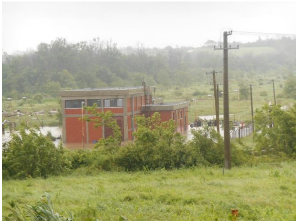
Water intrusion into the facility from which water is pumped out from the retention Kladnica
