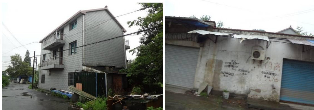
Figure 2-2 Residential Houses Constructed by AHs
