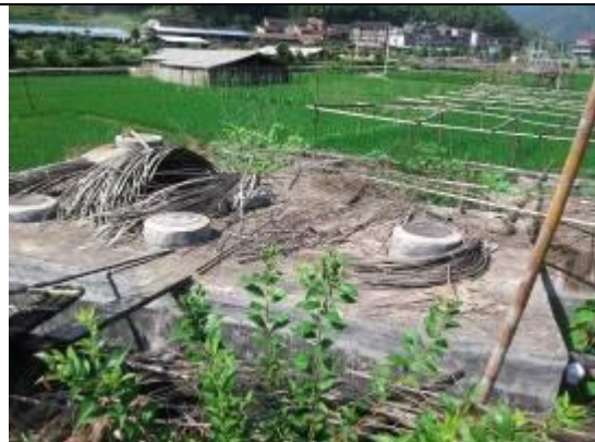
Site for WWT tank in Xiaohuangnan
