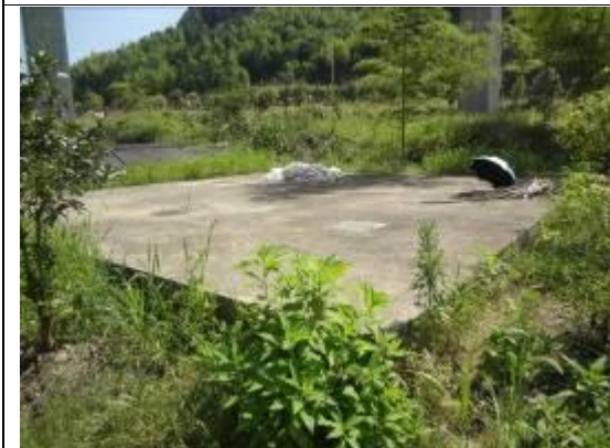
Site for WWT tank in Jiba/Shangwu
