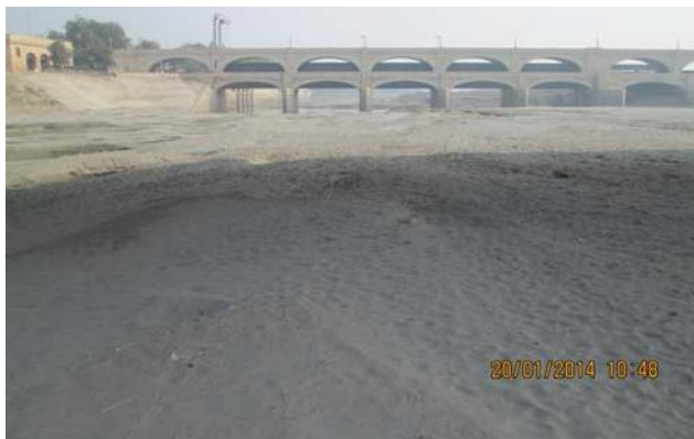
Downstream of Barrage during Closure 2014
