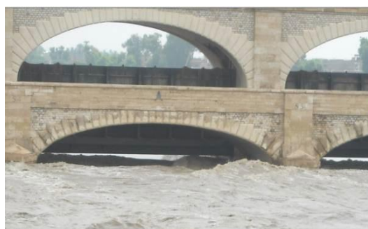
The underside of the masonry coping on the cutwater is 202.5. The flow water appears to be lapping up to this level.
