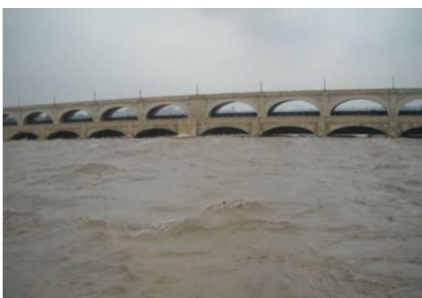
The water surface is close to underside of fully open gates, approximately 300mm clearance.
