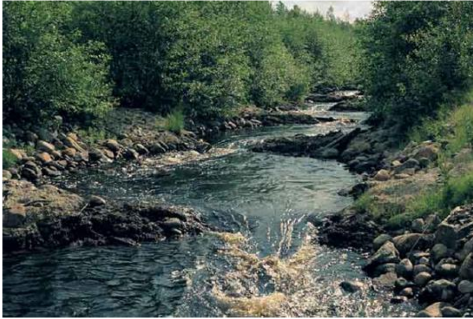
Figure 8-2 Nature Imitation Fish Pass
