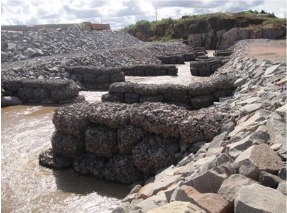
Gabion-type fishway
