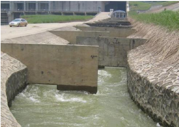
Fishway side wall with grouted rubble material
