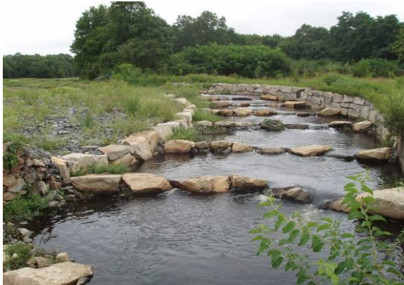
Enrockment-type nature-like fish passage
