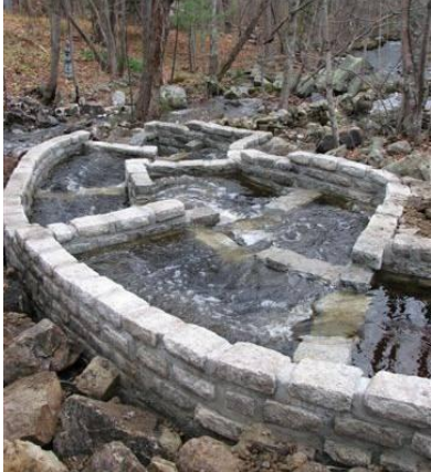
Reinforced grouted rubble nature-like fish passage
