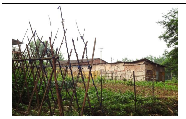
Figure 2-1 Photos of houses to be demolished
