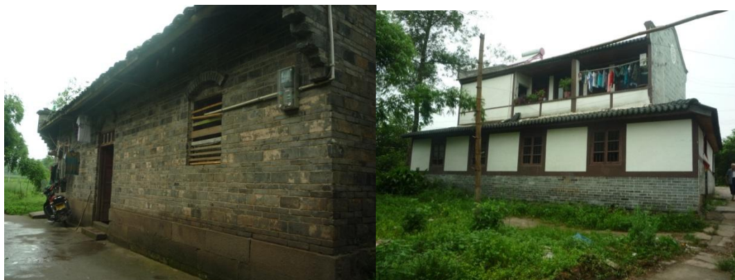
Figure 2-1 Photos of Houses to be Demolished
