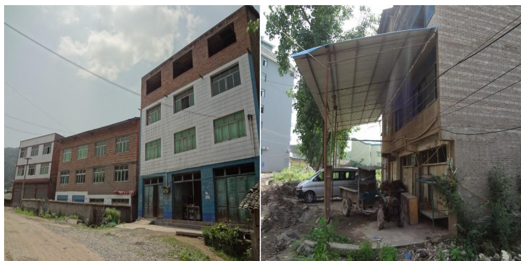
Figure 2-1 Photos of Houses to be Demolished
