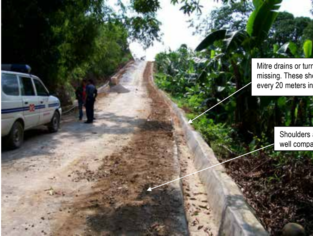
FMR above is provided with paved carriageway along steep gradient. (CMARPRP)
