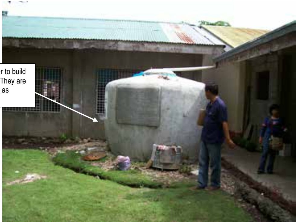
Ferro-cement water tank for rainwater collection.
