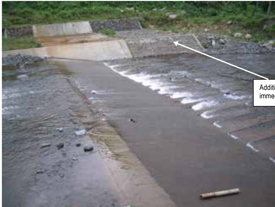
Slope protection built immediately upstream of the dam.
