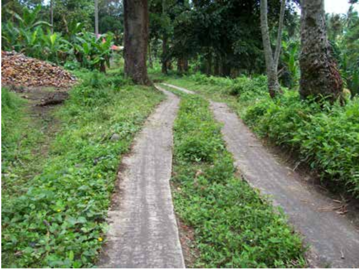
In some cases a concrete tire path may be a more practical alternative design for rural roads. (ASFP)
