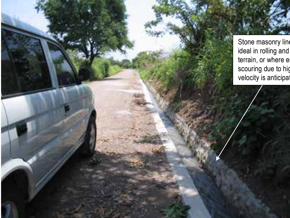
FMR with concrete/stone masonry lined canal. (ARCDP2)
