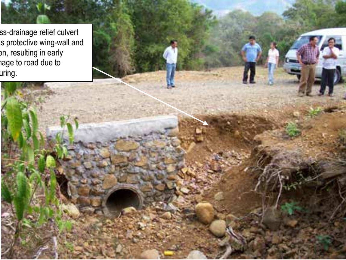
Poorly designed drainage structure. (MRDP1)
