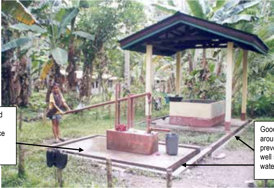
Single point system (deep well) with Laundry Tub and Shed
