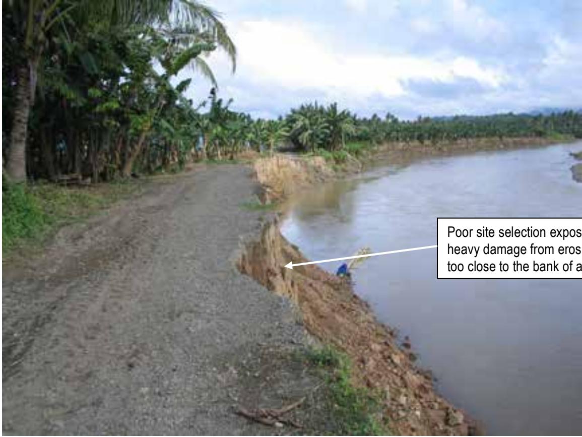
FMR damaged due to scouring.
