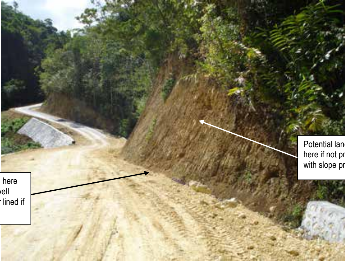
Damage on the road carriageway due to poor drainage. (ARCDP2)
