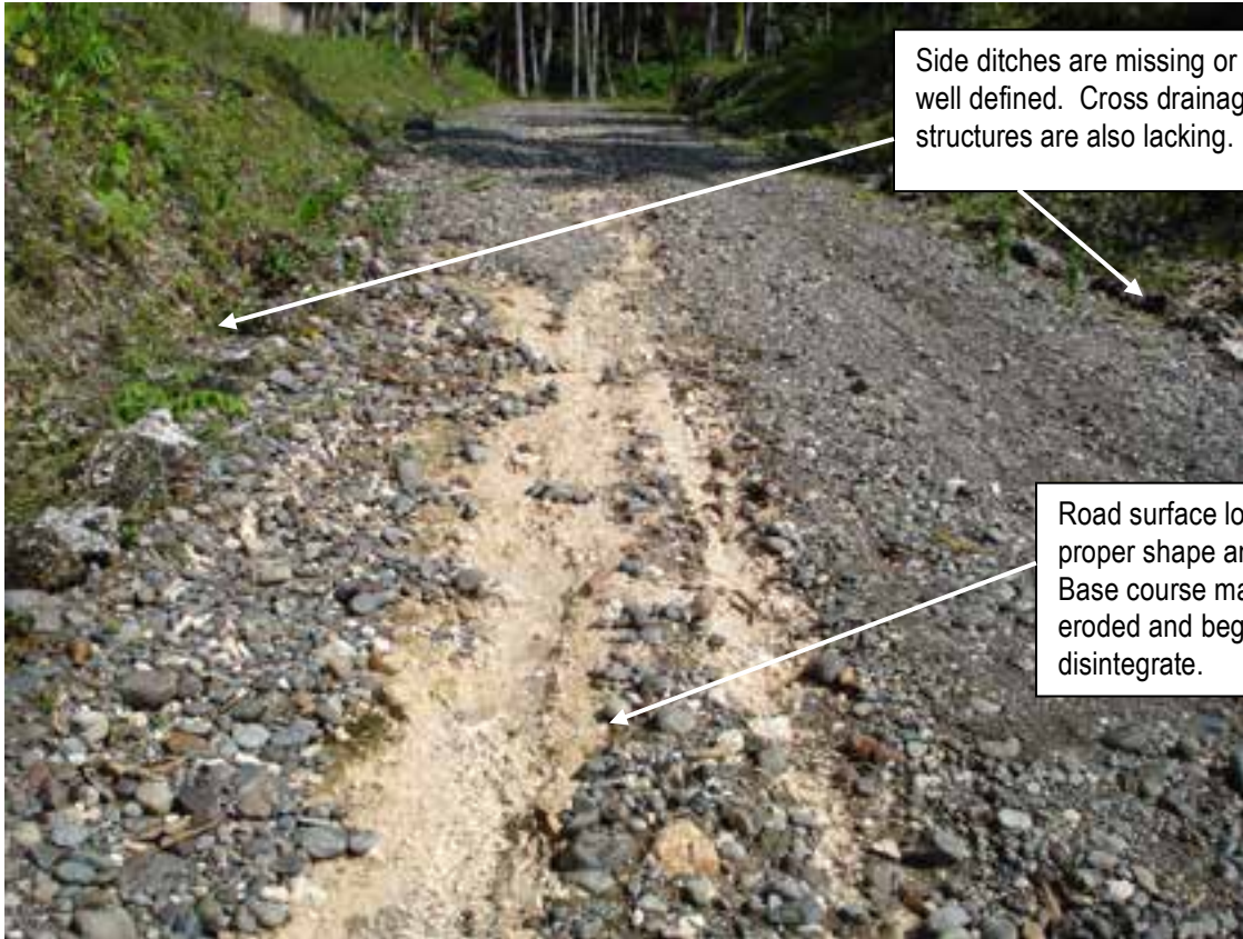
Damage on the road carriageway due to poor drainage. (ARCDP2)
