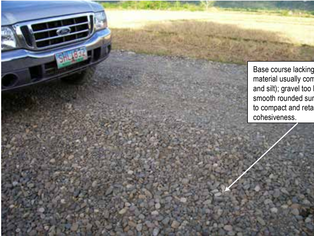
Road surface is not according to specifications. (ARCDP2)
