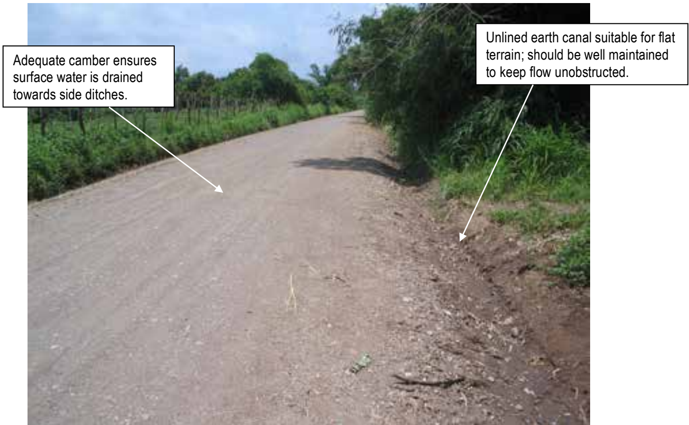
Well constructed, well drained road with unlined earth canal. (ARCDP2)
