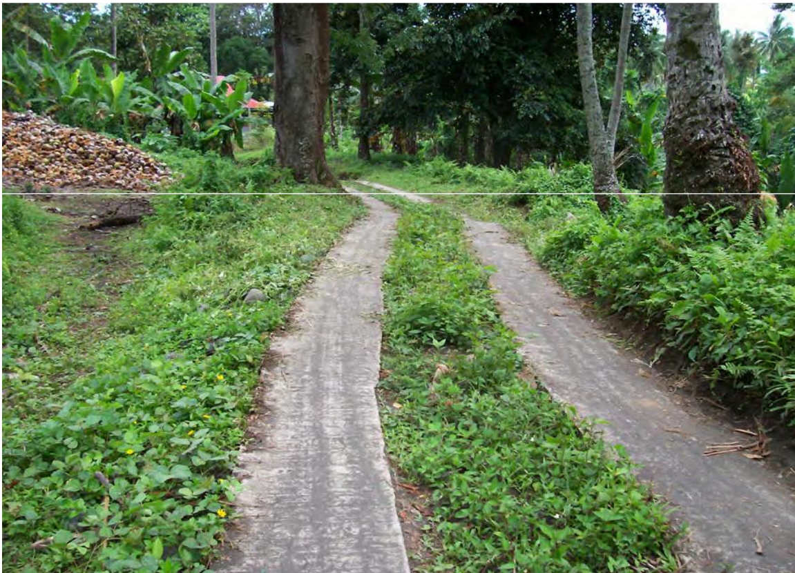
In some cases a concrete tire path maybe a more practical alternative design for rural roads. (ASFP)
