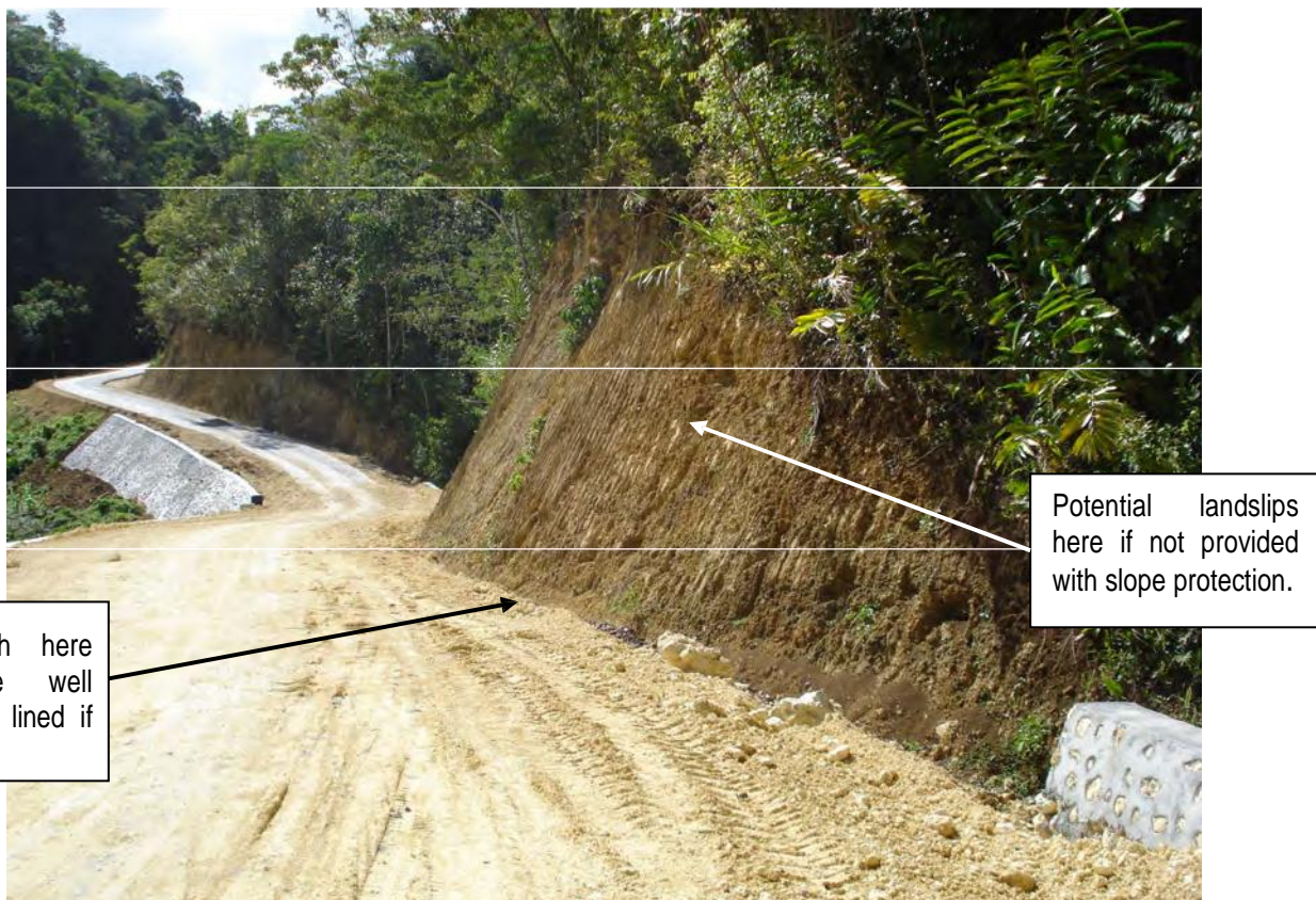
Damage on the road carriage way due to poor drainage.(ARCDP2)
