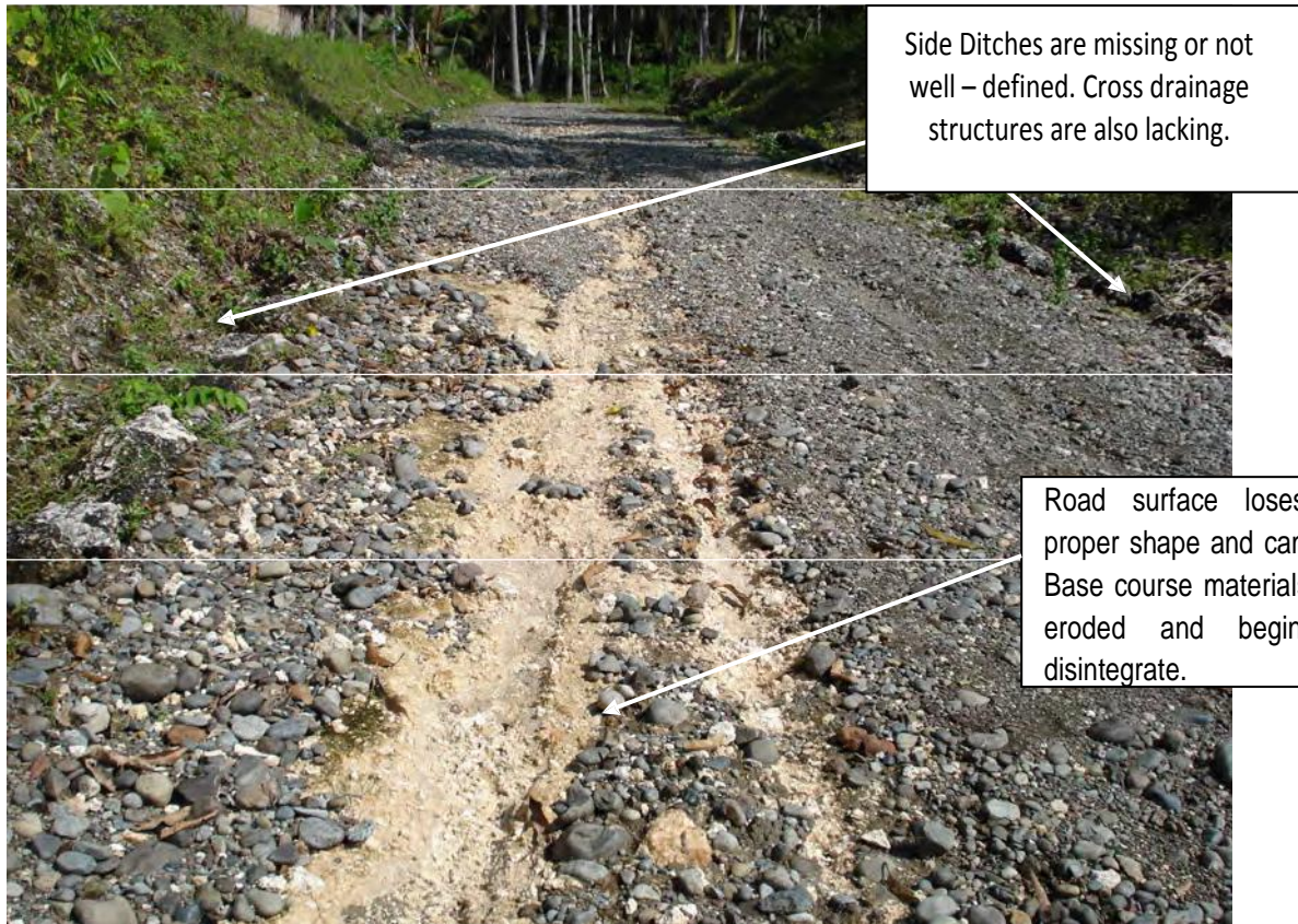
Damage on the road carriage way due to poor drainage.(ARCDP2)
