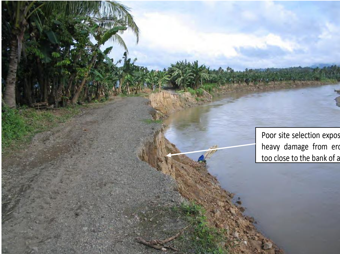
FMR damaged due to scouring
