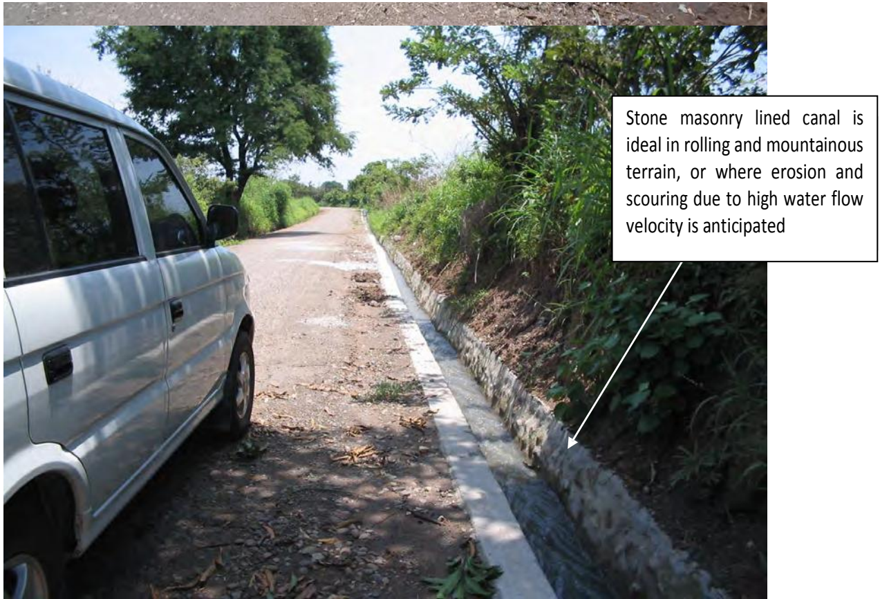
FMR with concrete/stone masonry lined canal. (ARCDP2)
