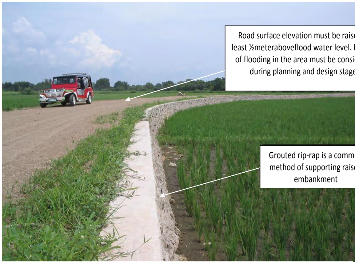
FMR with raised embankment supported by concrete stone masonry or grouted rip-rap retaining walls. (ARCDP2)
