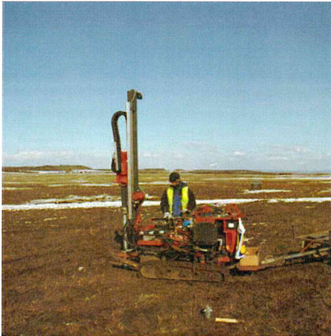
Construction of PVP
