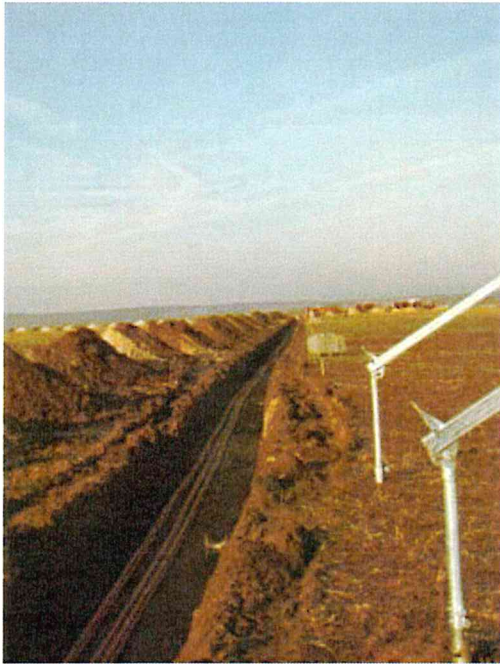
Construction of PVP
