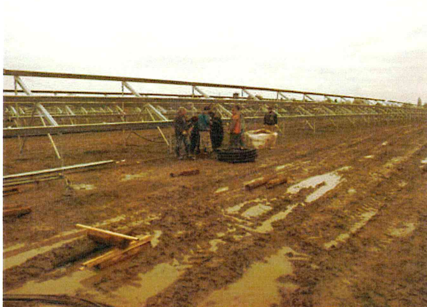
Construction of PVP
