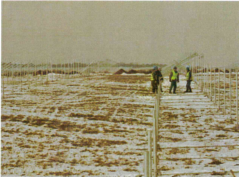
Construction of PVP
