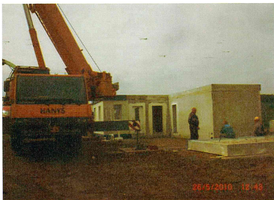
Construction of PVP
