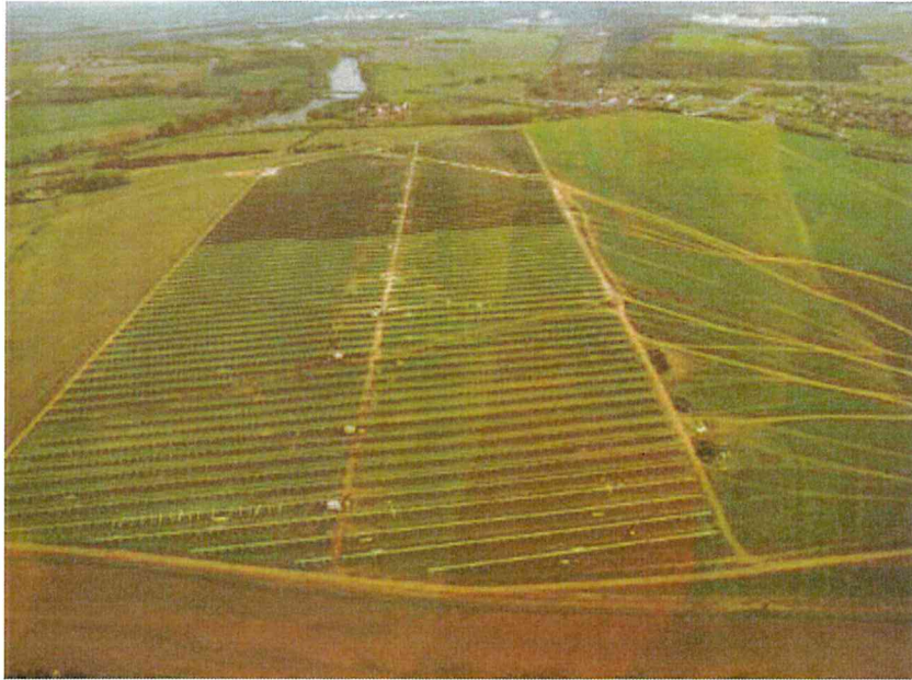
Construction of PVP
