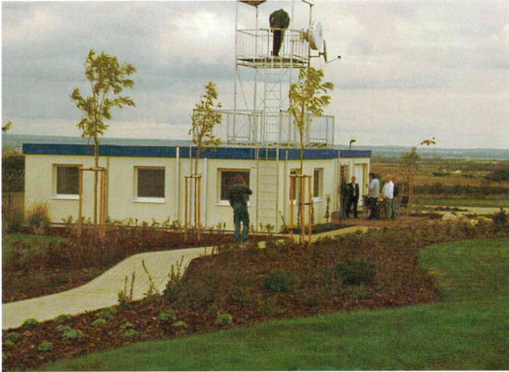
Control center after having finished all works
