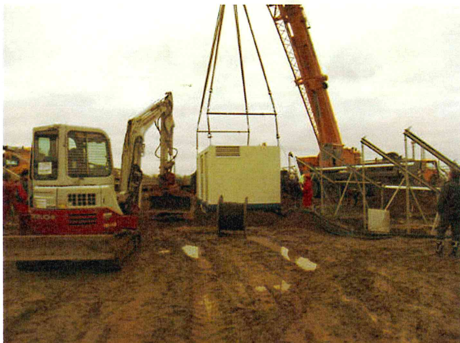
Construction of PVP
