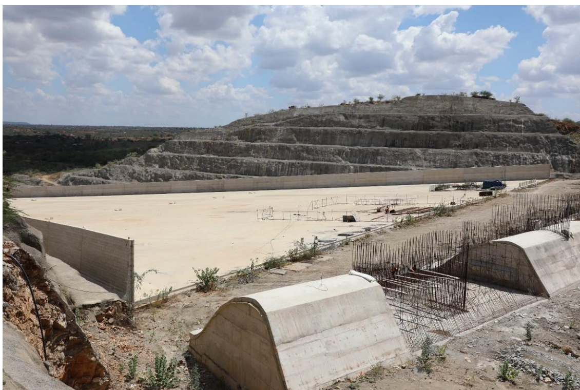
Figure 14 A View of Thwake Dam Spillway ongoing works /Picture/Courtesy/PIT
