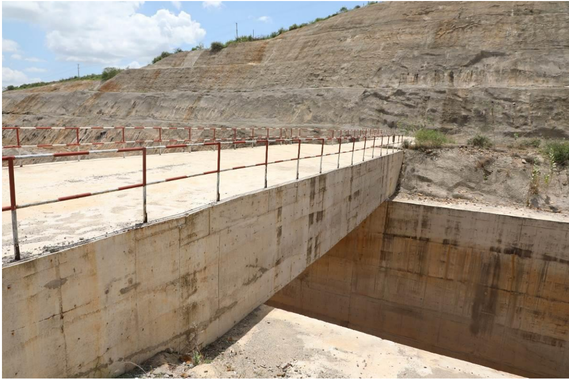
Figure 17 A section of a concrete footbridge near the tunnels /Picture/Courtesy/PIT
