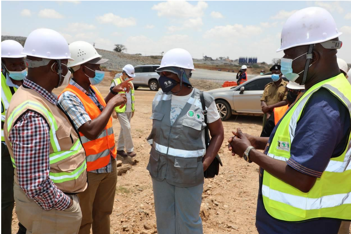
Director General, AfDB Regional Development and Business Delivery Office with other Bank officials during a site inspection visit on March 9, 2022/Picture/Courtesy/PIT
