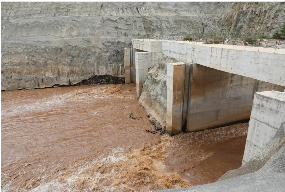
Figure 16 A view of the tunnels with water flow (December 2024) /Picture/Courtesy/PIT
