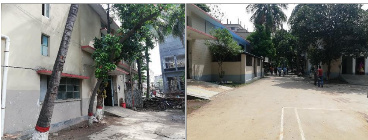
Figure 5: Existing Condition at the BITAC Site
