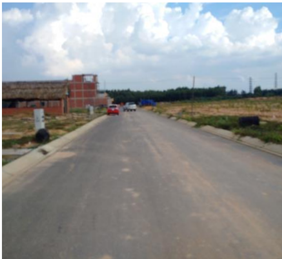
Infrastructure in Phuoc Thien resettlement site (phase 1)
