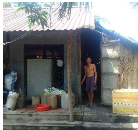
House of Mr. Bui Thanh Hiep in Long Hieu Hamlet, Long Tan Commune affected by Project
