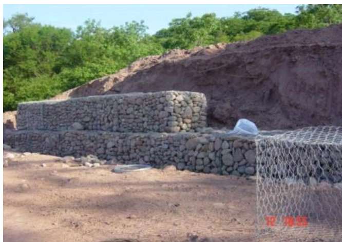
Photograph 4.3: An Example for Gabion Wall
