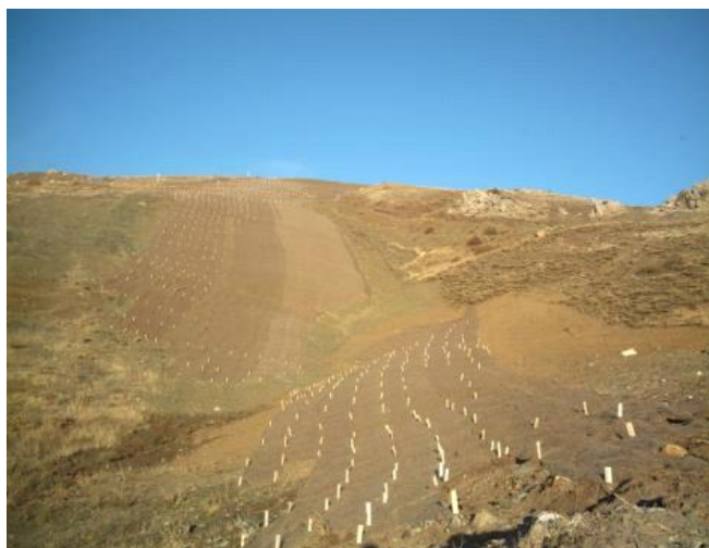
Photograph 4.4: An Example for Erosion (Jute) Matting
