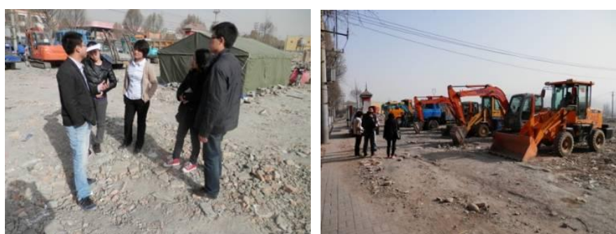
Figure 4-2 Construction Site of the Resettlement Community
