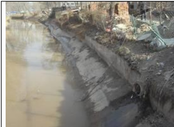
Wastewater discharge in a canal
