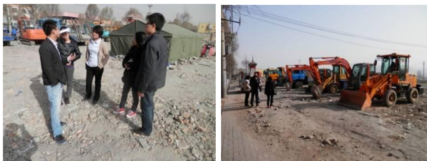
Figure 3-2 Construction Site of the Resettlement Community
