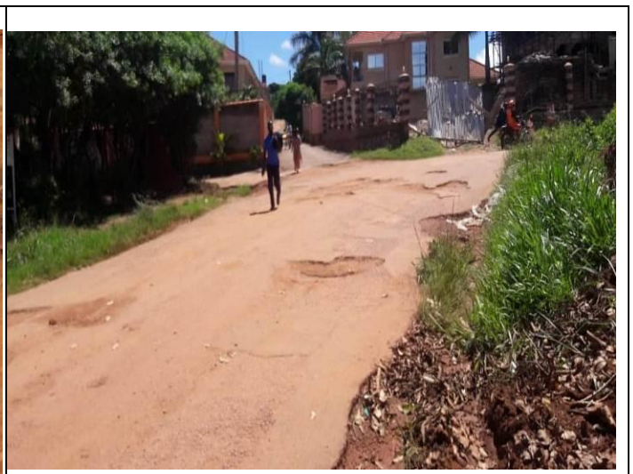
Plate 4: Uneven road surface with potholes along Luwafu road
