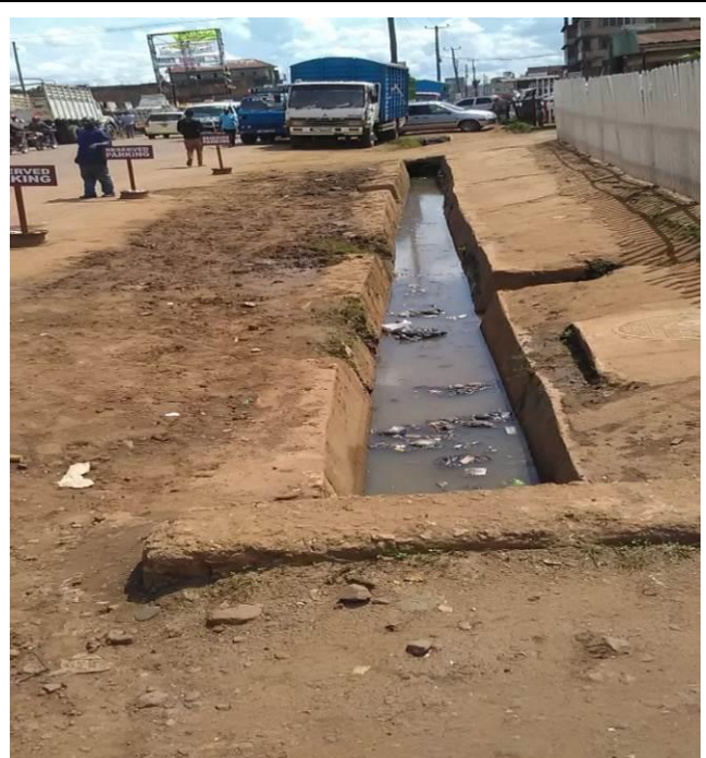
Plate 6: Silted trench in Ndeeba along Kibuye-Busega Road
