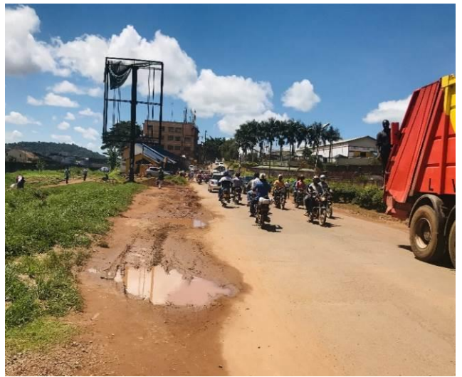
Plate 8: Worn out road shoulders along the Eighth Street Road
