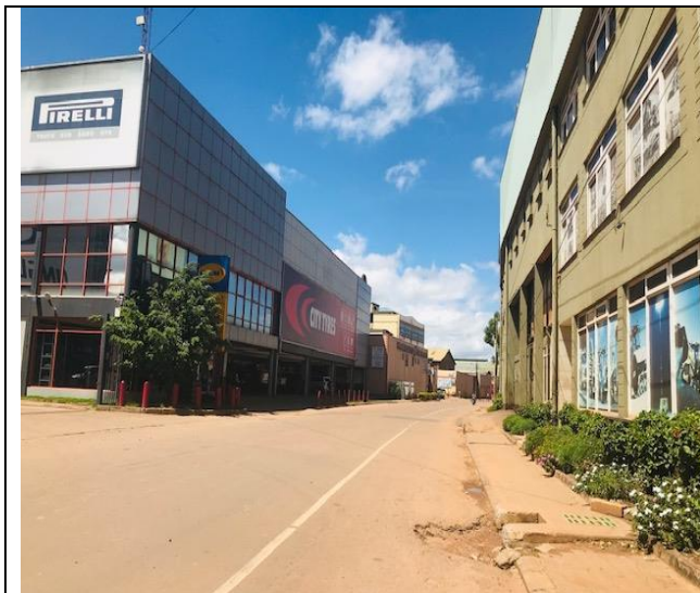
Plate 1: Buildings Close to Carriageway along Sixth Street Road
