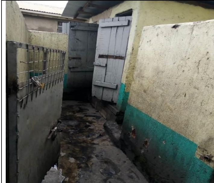
Plate 3: Poor Excreta Facility, Kitintale Market along Portbell road
