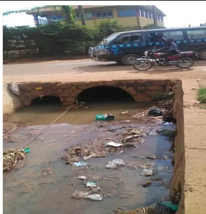
Plate 5: Blocked drainage channel along Kibuye-Busega Road
