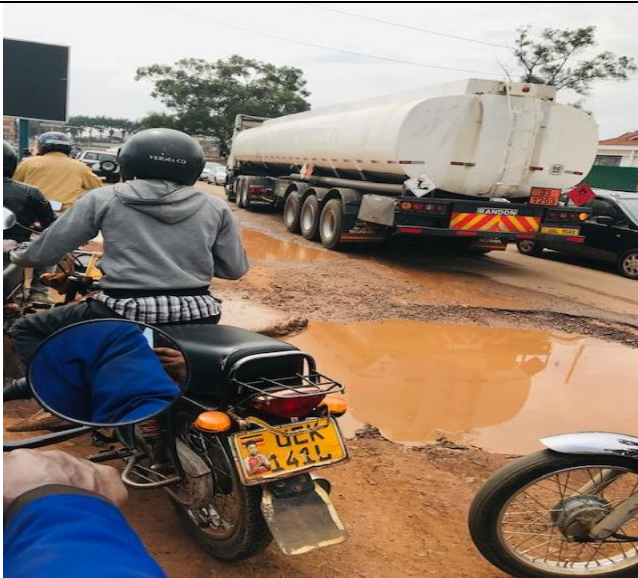
Plate 11: Flooded pothole within the carriage along Eighth street Road
