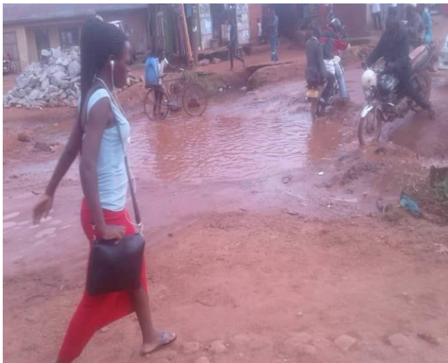
Plate 7: Waterlogged pothole along Ssuna Road (Diniya Mosque)
