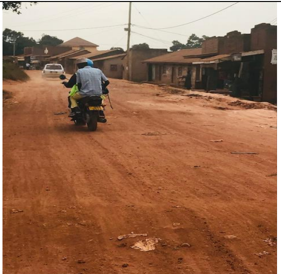
Plate 2: Road condition of Murrum roads (Mugema road)
