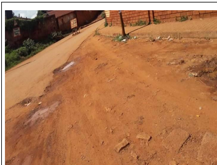
Plate 3: Inadequate extension of tarmac to connecting roads along Luwafu road
