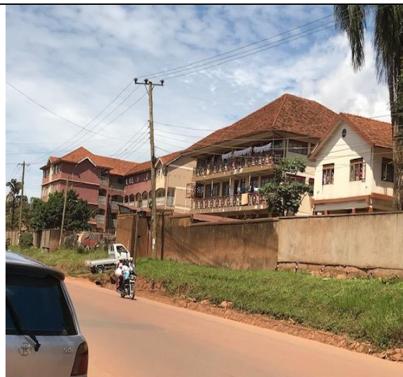
Plate 2: S Sir Apollo Kaggwa Primary School Close to the Road along Sir Apollo Kaggwa Road
