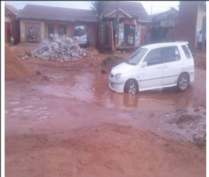
Plate 12: Flooded pothole within the carriage way along Ssuna road
