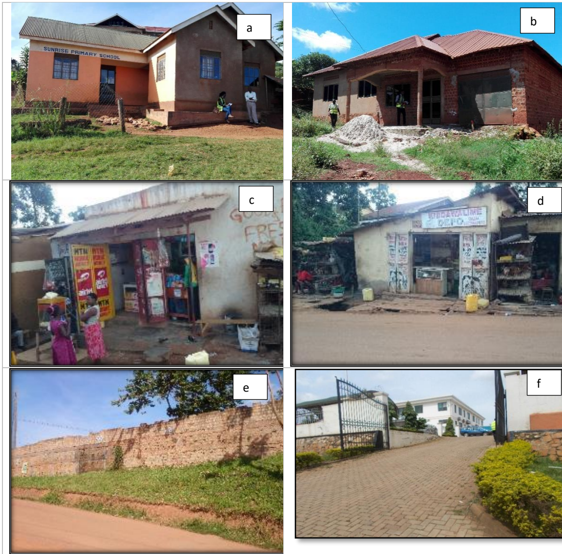
(a) Residential structure serving as a Nursery School along Kabuusu-Kitebi-Bunamwaya road, Seguku Zone 5, Chainage 1+210
