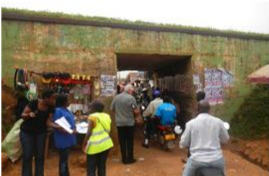
Plate 17: The underpass structure under the railway line
