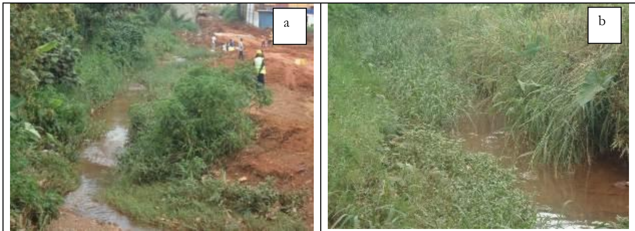
Plate 8: Stream by Nakawa –Ntinda road: (a) On-going construction by the stream; (b) Plant species by the stream
