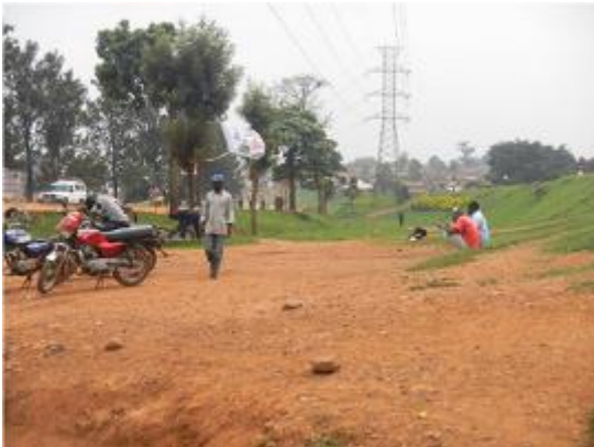
Plate 20: The railway embankment on the right, the 132kV Transmission line, and Queen's Way to the left
