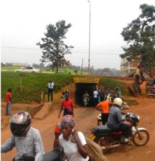
Plate 16: The underpass structure under Queens Way
