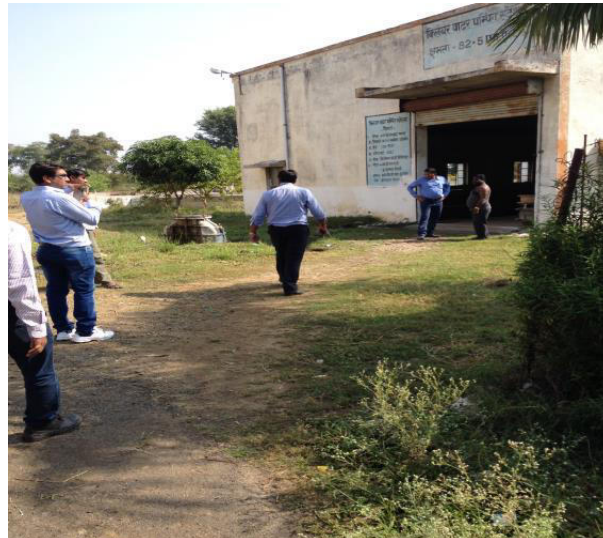
Existing WTP near Rajghat Dam
