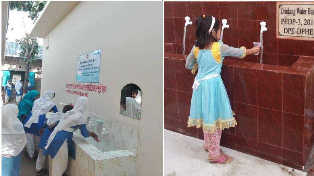
Figure 18: Multiple user Hand Washing System
