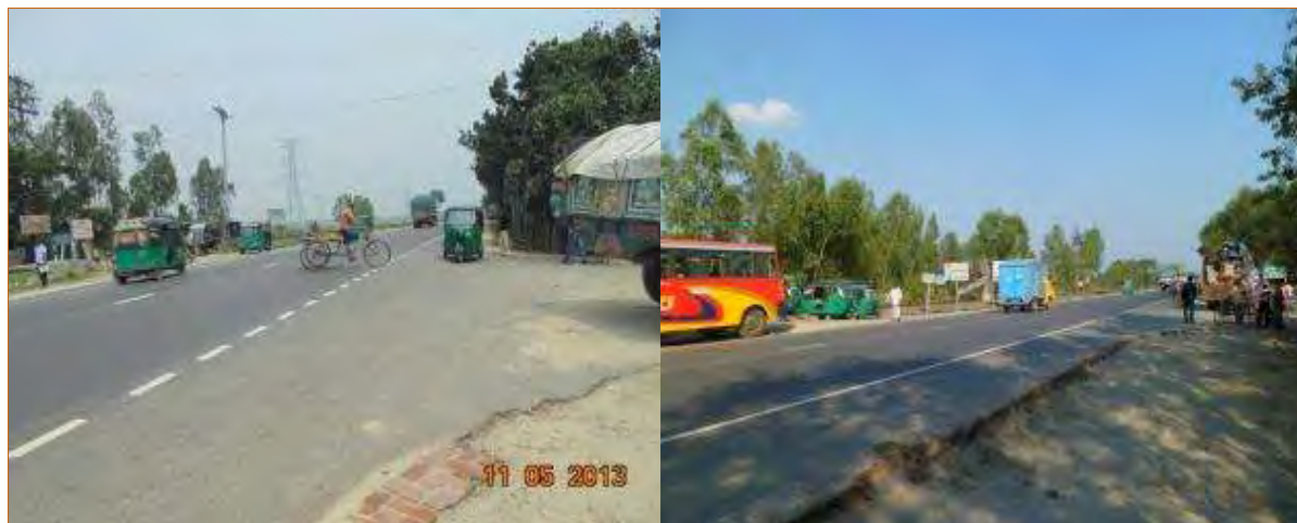
Photograph 9: Dangerous Road Crossing at Elenga-Hatikamrul Road
