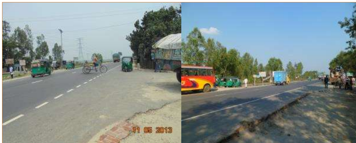
Photograph 9: Dangerous Road Crossing at Elenga-Hatikamrul Road
