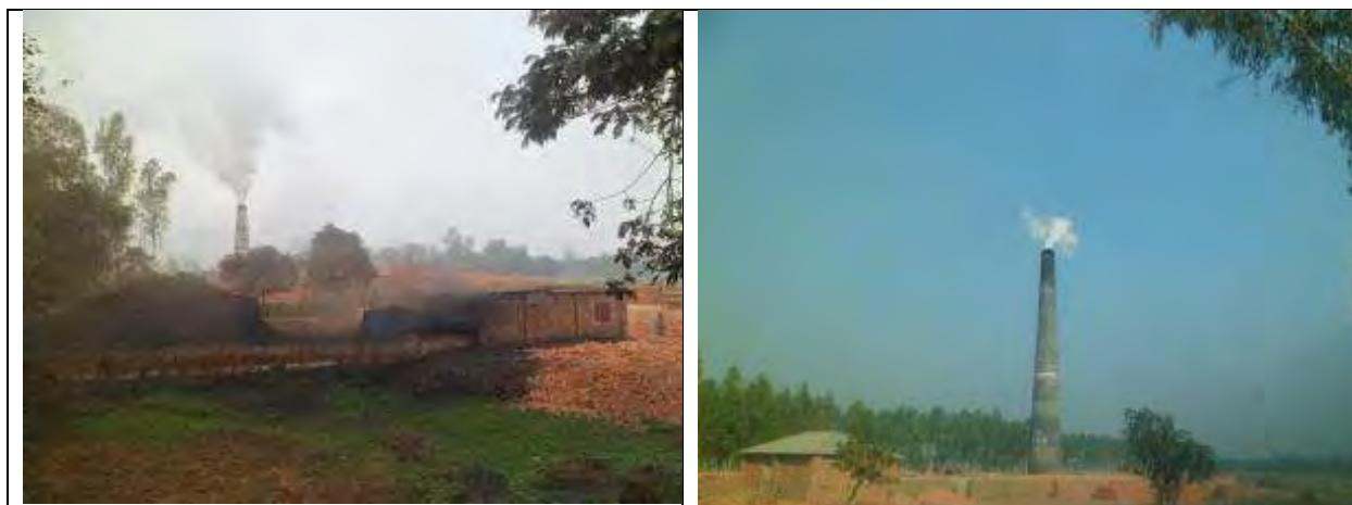
Photograph 6: Sources of Air Pollution along the Hatikamrul-Rangpur Road
