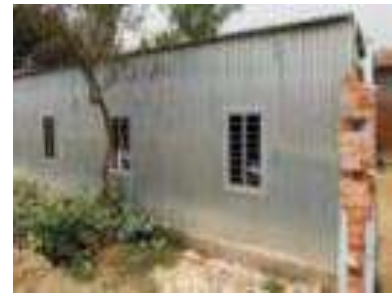
Right picture: A temporary school made of galvanized iron sheets has been constructed, while the concrete school building is not yet finished.
