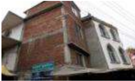
Left picture: The existing mosque which has a pending issue on ownership located in Hatubanga, Gorai, Tangail district
