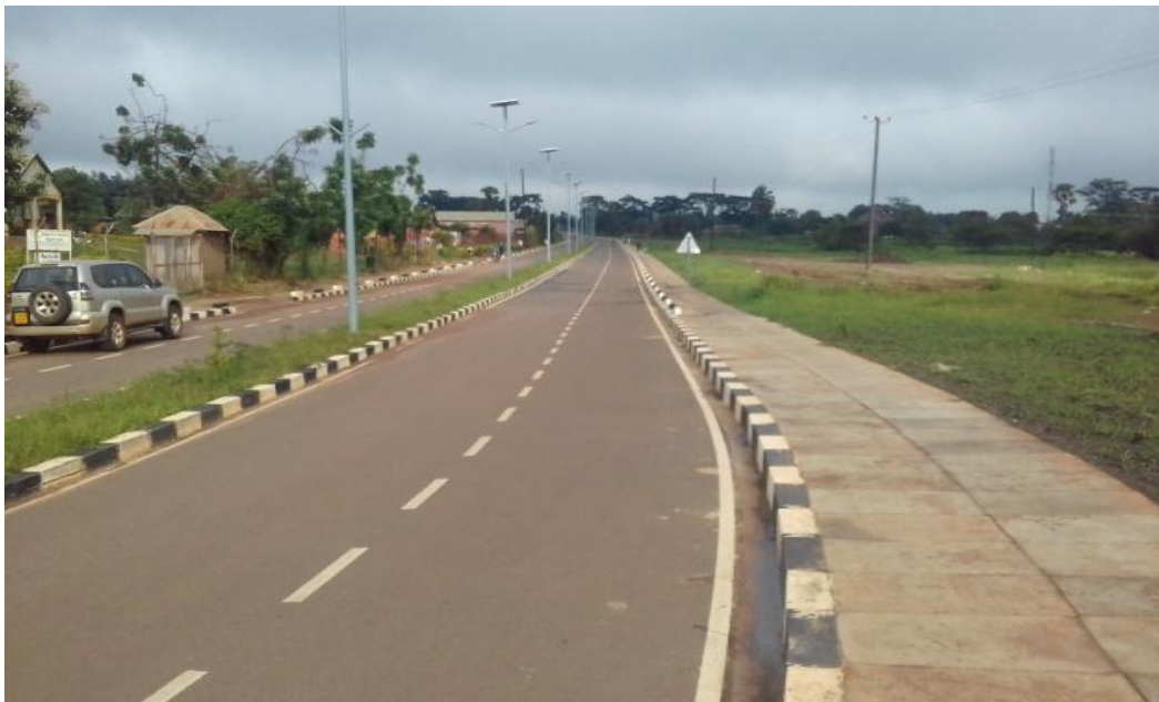
Commercial Road under USMID in Gulu (After)
