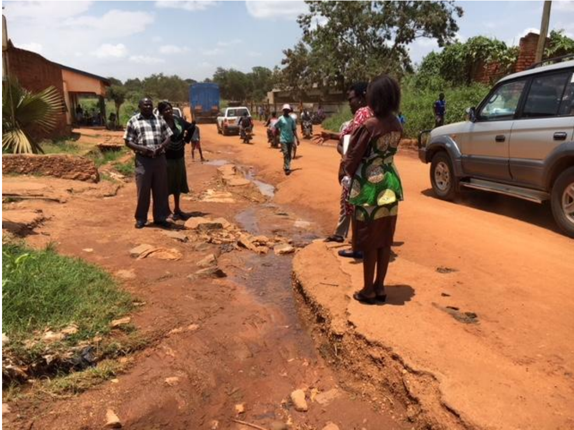
Lack of drainage system and road erosion in Kitgum
