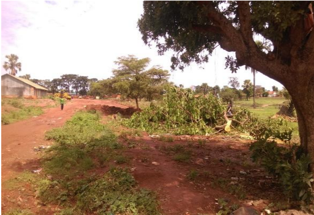
Commercial Road under USMID in Gulu (Before)
