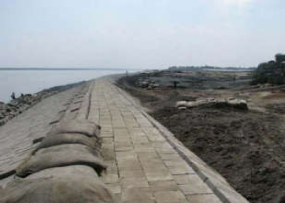
Figure 4-16 Photograph 2007 Old Embankment Newly Re-Constructed with Cement Blocks
