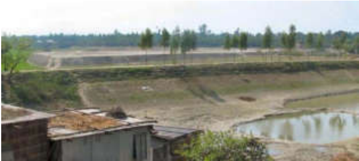
Figure 4-22 Photograph of Old Embankment Resettlement Village Platform near Completion, Dry Season 2006
