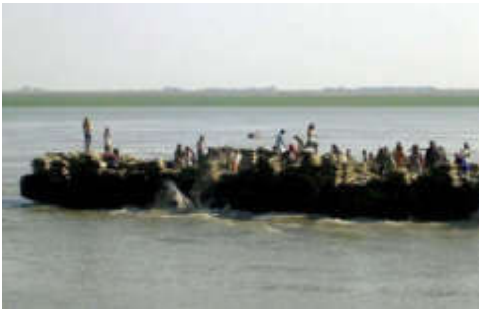
Figure 4-13 Photograph of Primary Protection through Systematically Dumped Geobags from Barge
