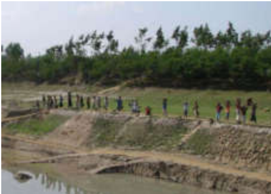
Figure 4-21 Photograph of Old Embankment Resettlement Village Construction, Dry Season 2006
