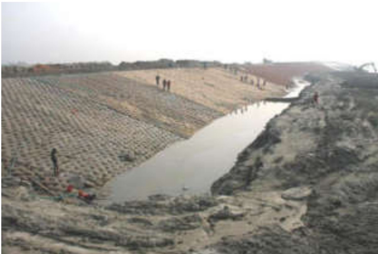
Figure 2-6 Installation of grout-filled jute mattress (Harirampur Feb 2019)
