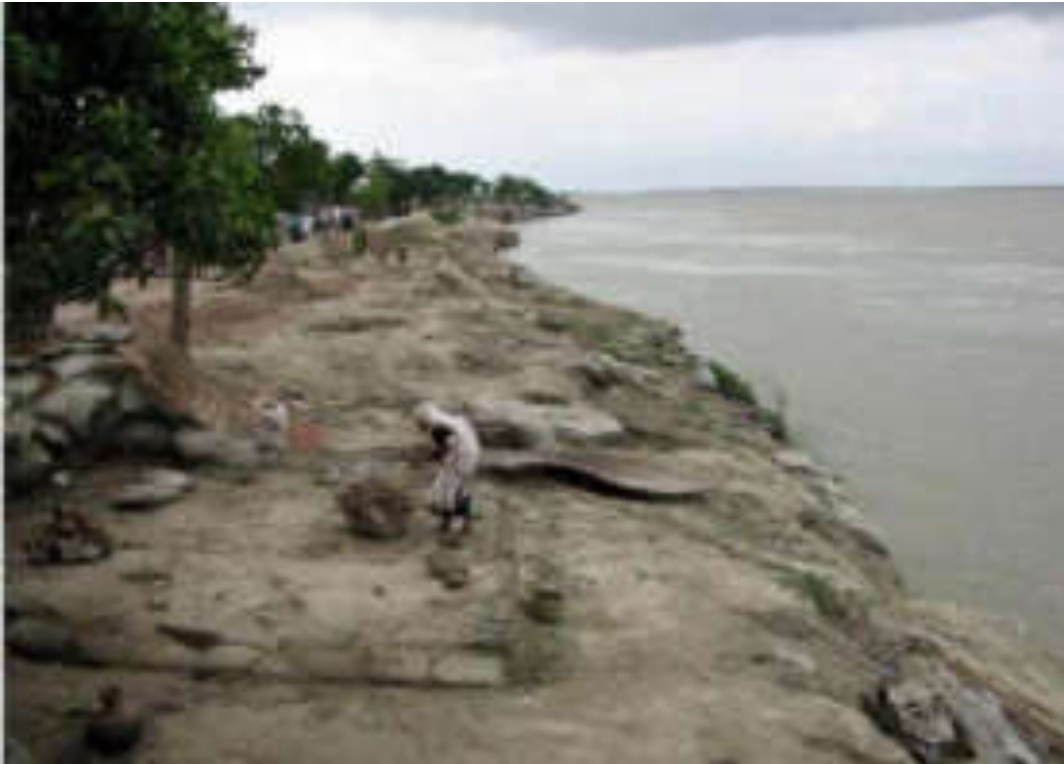
Figure 4-9 Photograph, Results of Bankline Erosion
