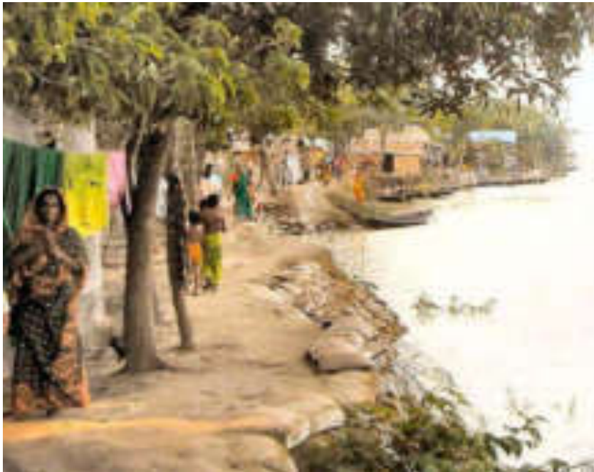
Figure 4-25 Old Embankment Villagers Prior to River Erosion Mitigation Work, 2003
