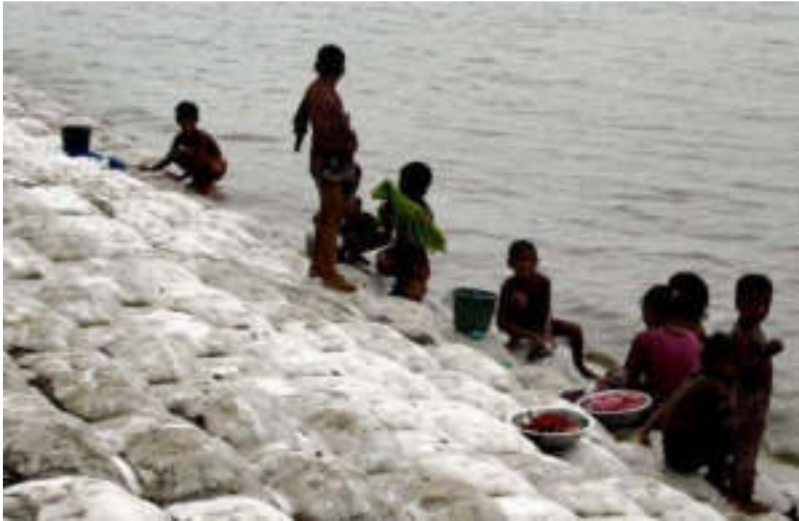
Figure 4-20 Photograph 2007 Old Embankment Finished Permanent Protection with Cement Filled Mattress
