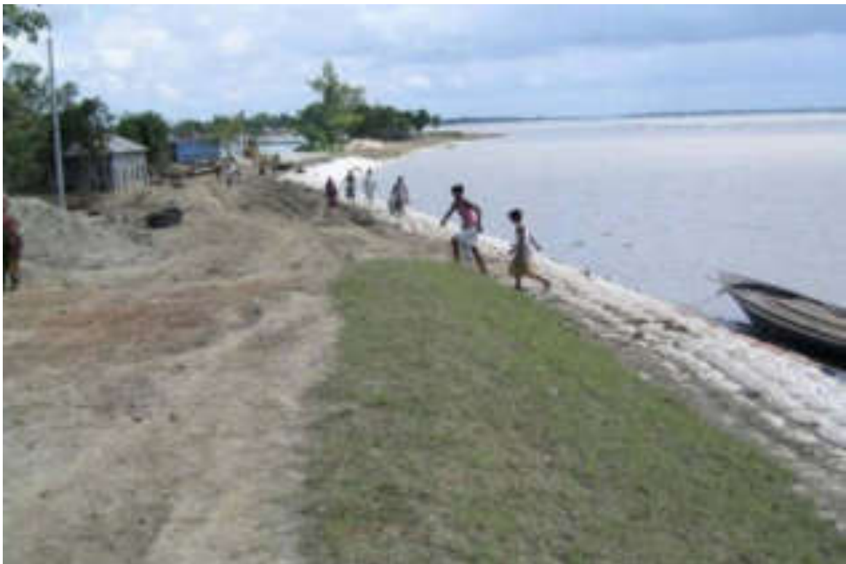
Figure 4-15 Photograph 2007 Old Embankment after Community Resettled and Final (Underwater) Protection Completed
