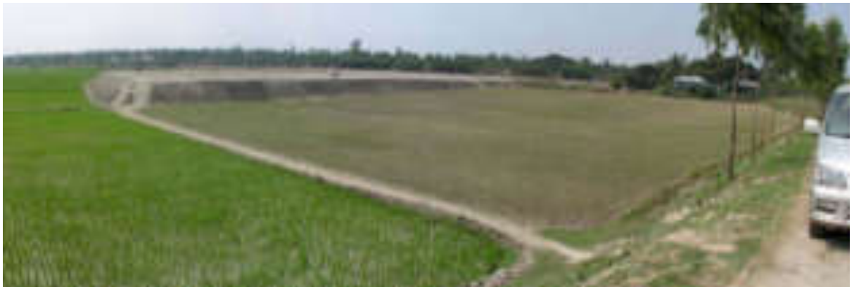
Figure 4-23 Photograph of Old Embankment Resettlement Village Platform near Completion, Dry Season 2006
