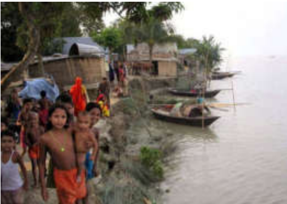
Figure 4-3 Old Embankment Village during Seasonal High Water Season, 2005
