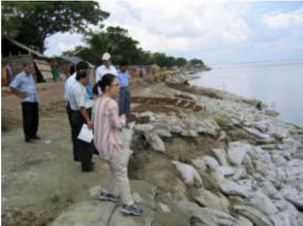
Figure 4-11 Photo of Geobag Temporary Protection along the Old Embankment
