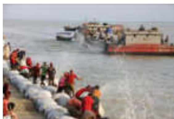
Figure 1-7 Dumping of Geobags
