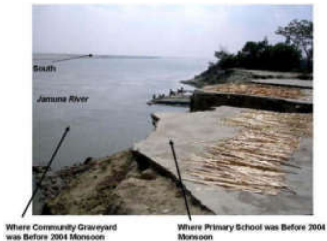
Figure 4-5 Location of Primary School and Grave Yard lost in 2004 Monsoon
