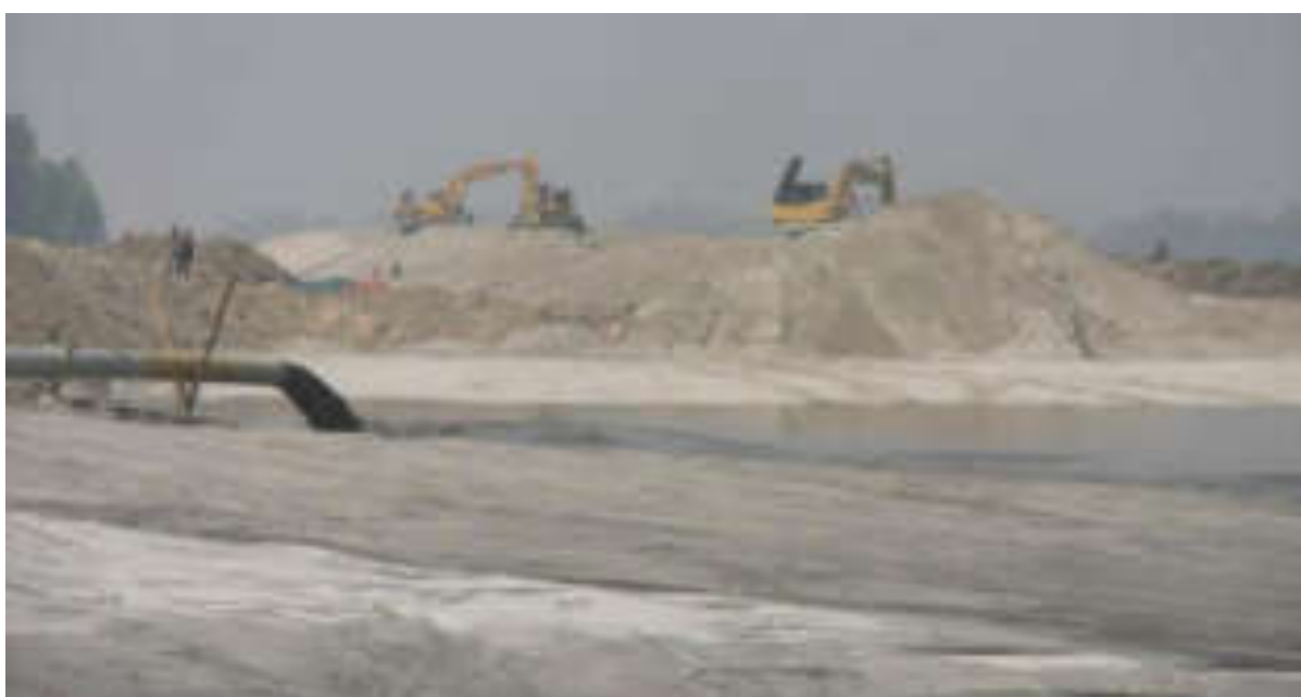
Figure 2-7 Embankment construction at JRB-1 with compacted dredged sand (Kaijuri, Feb 2019)
