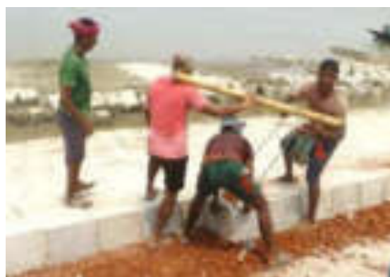
Figure 1-4 Placing of CC Blocks
