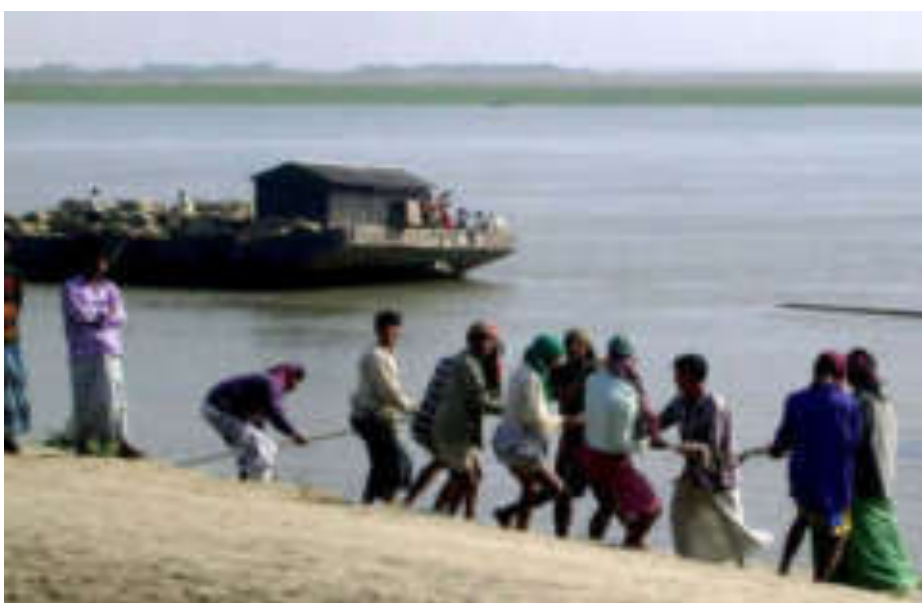
Figure 4-14 Photograph of Pulling Geobag Dumping Barge to a new Location
