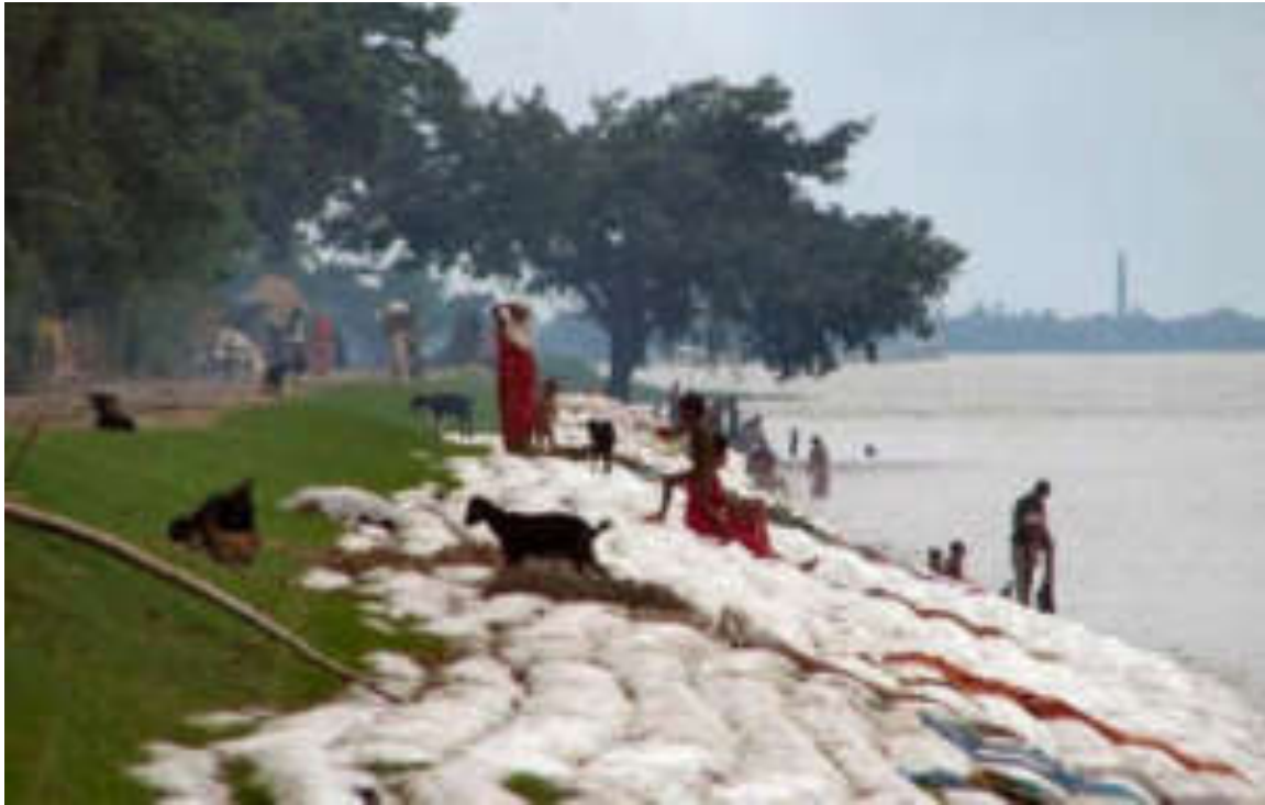
Figure 4-18 Photograph 2007 Old Embankment Finished Permanent Protection with Cement Filled Mattress
