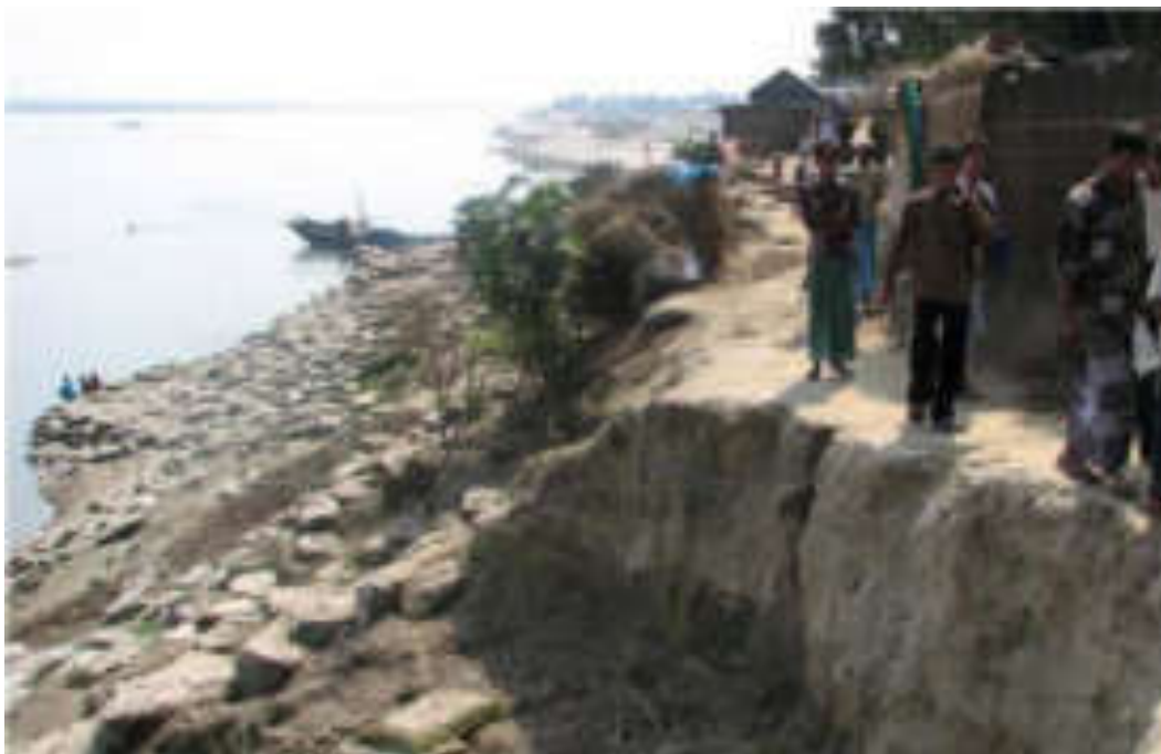
Figure 4-12 Photo of Geobag Temporary Protection along the Old Embankment
