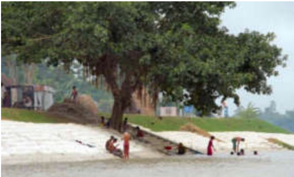
Figure 4-19 Photograph 2007 Old Embankment Finished Permanent Protection with Cement Filled Mattress
