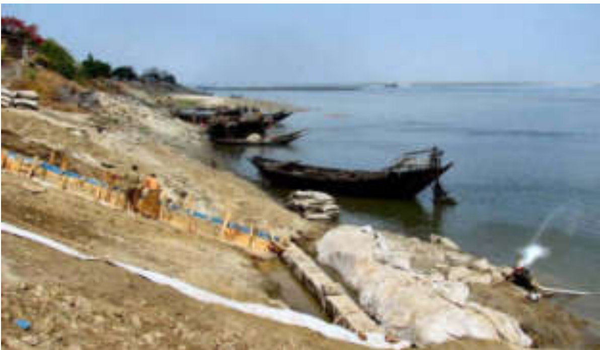
Figure 4-17 Photograph 2007 Old Embankment Preparing for Permanent Protection with Cement Filled Mattress
