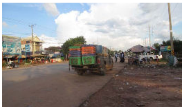
Road and drainage condition at NR6 section
