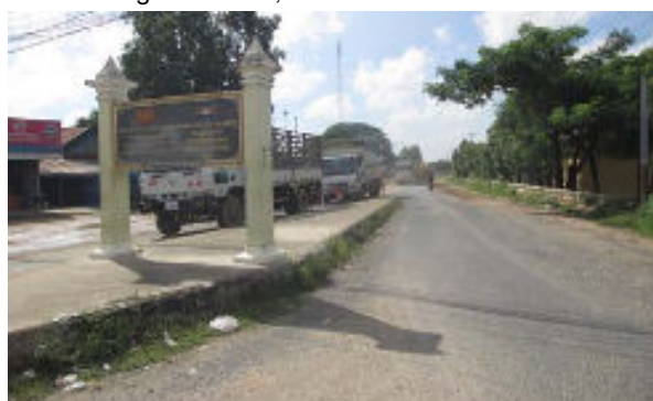
Intersection of NR1 with PR312
