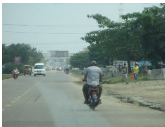
Traffic and road condition at NR1
