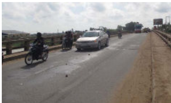
Existing bridge at Bour River in Preah Sdach district, Prey Veng province
