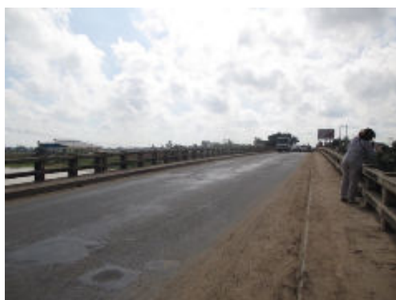
Existing bridge at NR1
