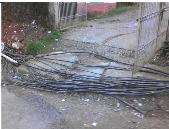
Existing spaghetti lines / household connections of water supply system in ward no 1, Ilam Municipality
