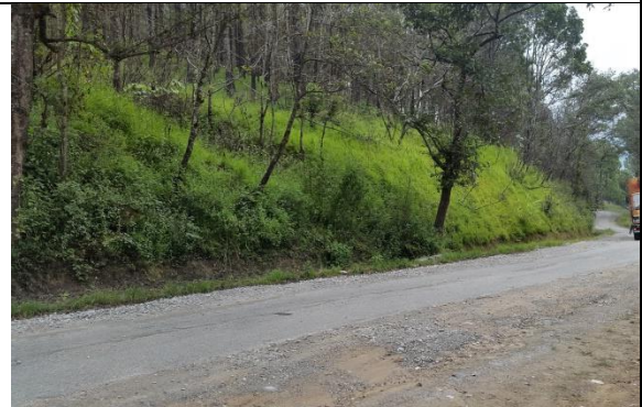
Access Road to the project location
