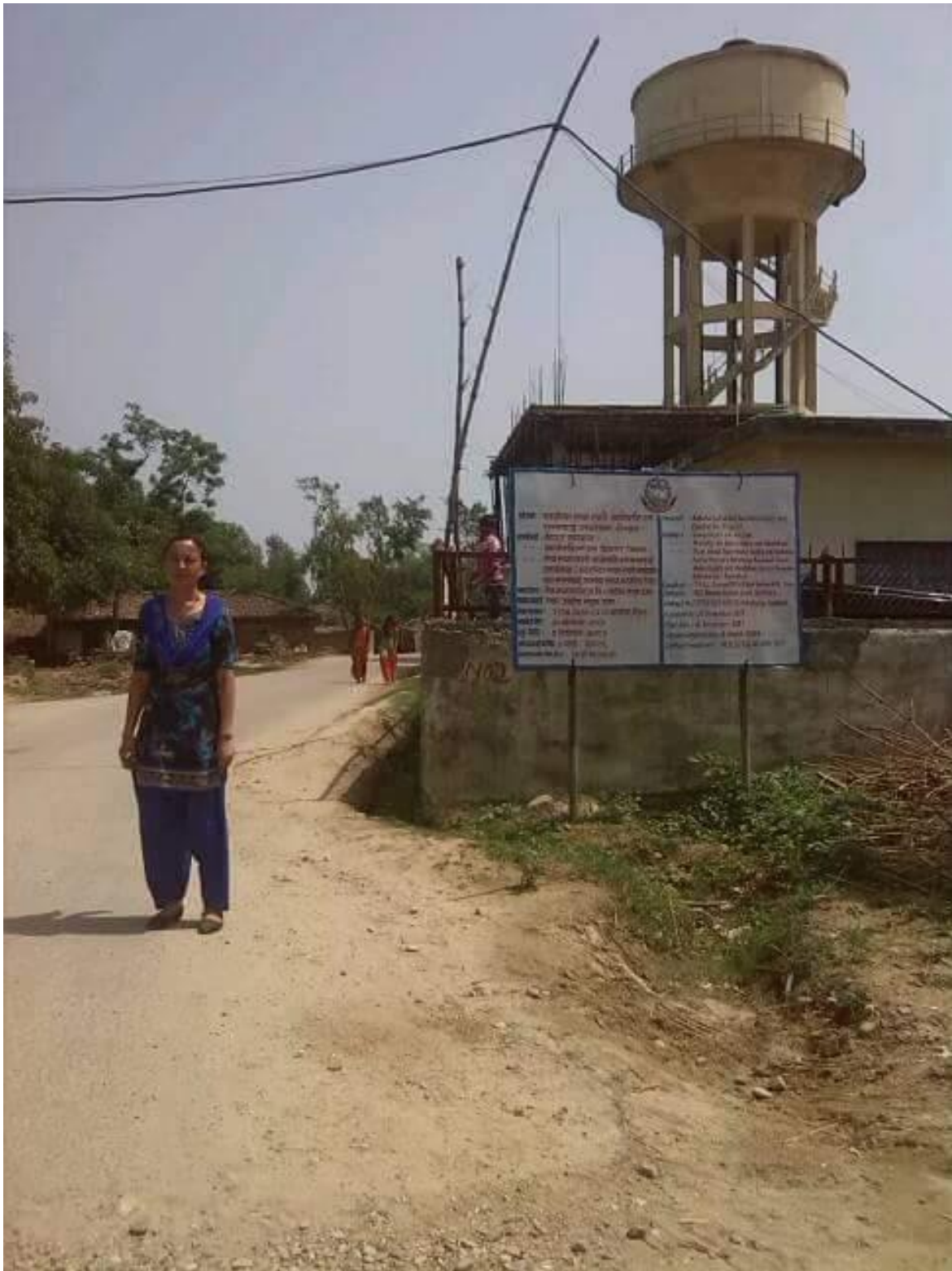
Figure 4: View of Drainage Starting Point
