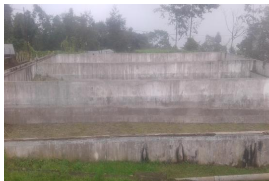
4. Non-functioning Existing Slow Sand Filter
