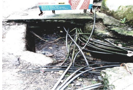
2. Existing condition of distribution pipelines
