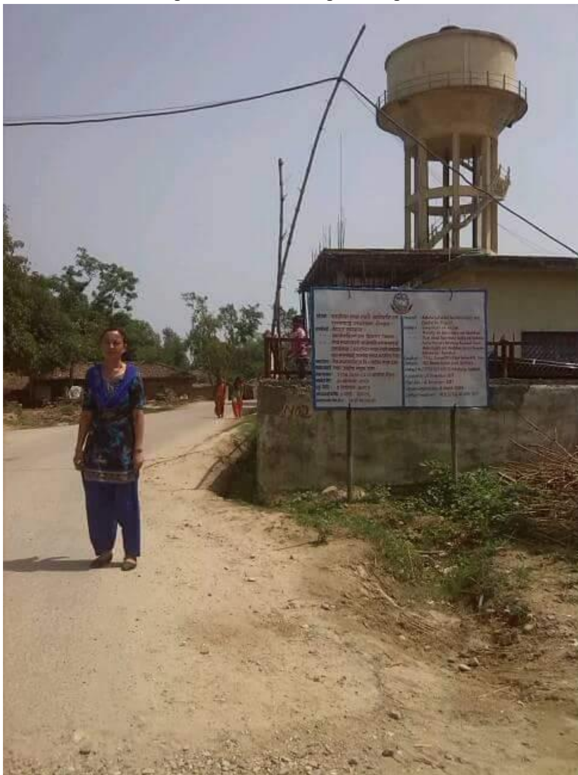
Figure 4: View of Drainage Starting Point
